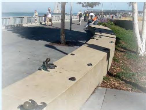
Seawall detail. Public art increases interest, encourages walking. Ledge provides walkers with a place to sit and rest. Ample width permits multiple streams, different speeds, strollers, families etc. San Francisco, California
