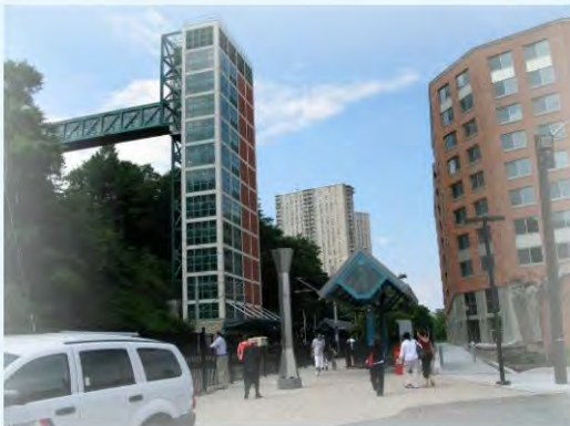
Elevator and pedestrian connection between two communities at different elevations. The connection has a dual use functioning as a community connector and direct access to transit. Hoboken, New Jersey
