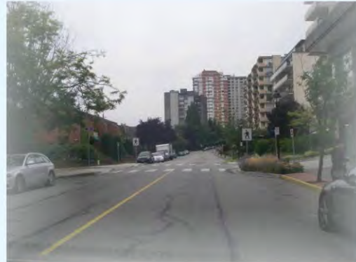
Pedestrian friendly crossing, 18th Street and Bellevue Avenue. West Vancouver, BC
