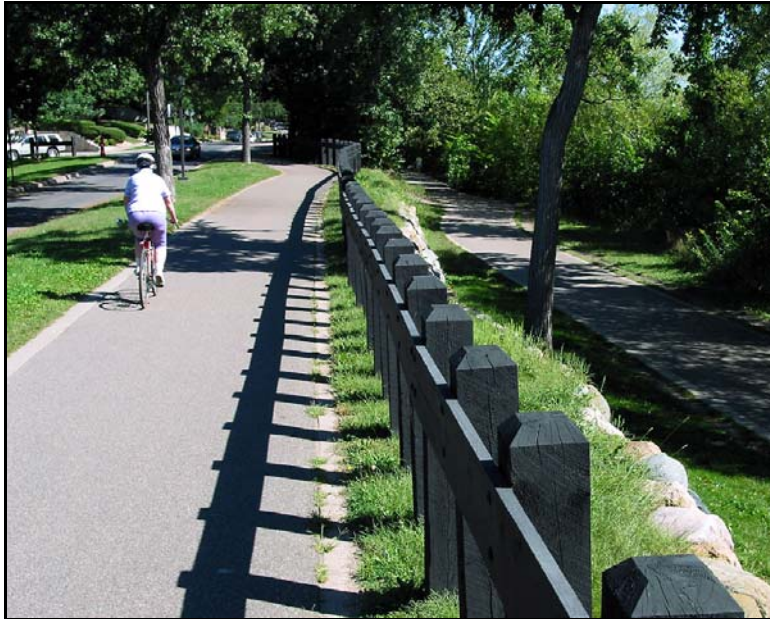
Figure 4.14 — Safety railing adjacent steep side slope
