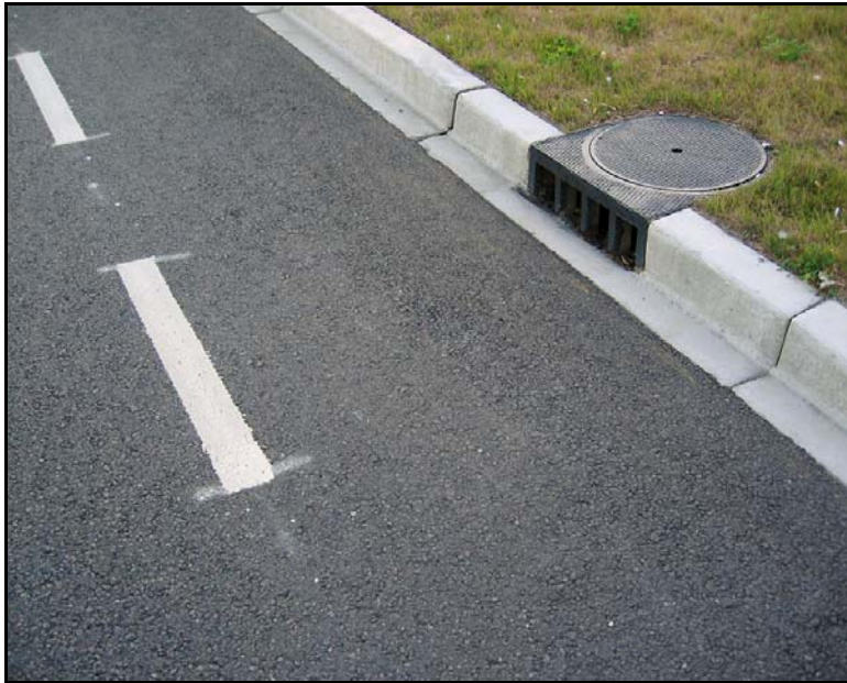
Figure 4.5 — Bicycle-friendly gutter and catchbasin
