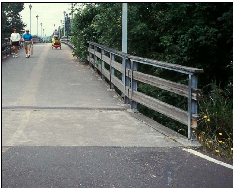
Figure 4.18 — Railing flared at bridge end
