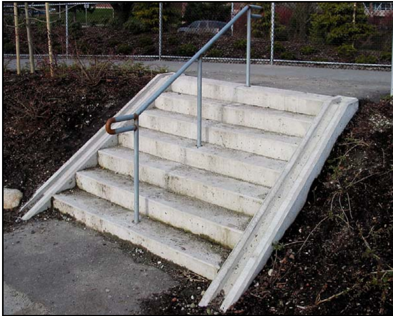
Figure 4.19 — Bicycle ramp on stairs
