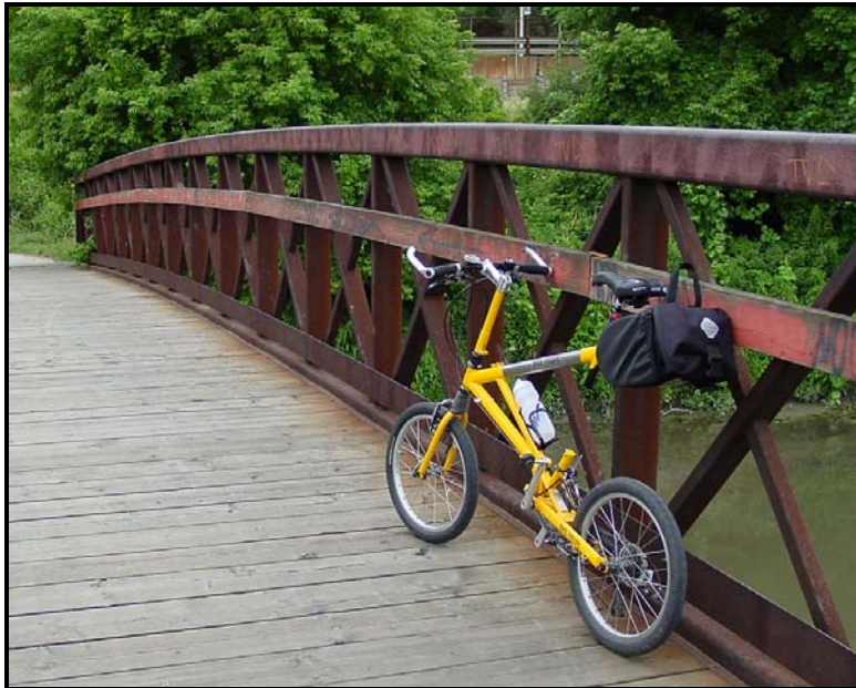
Figure 4.18 — Railing flared at bridge end
