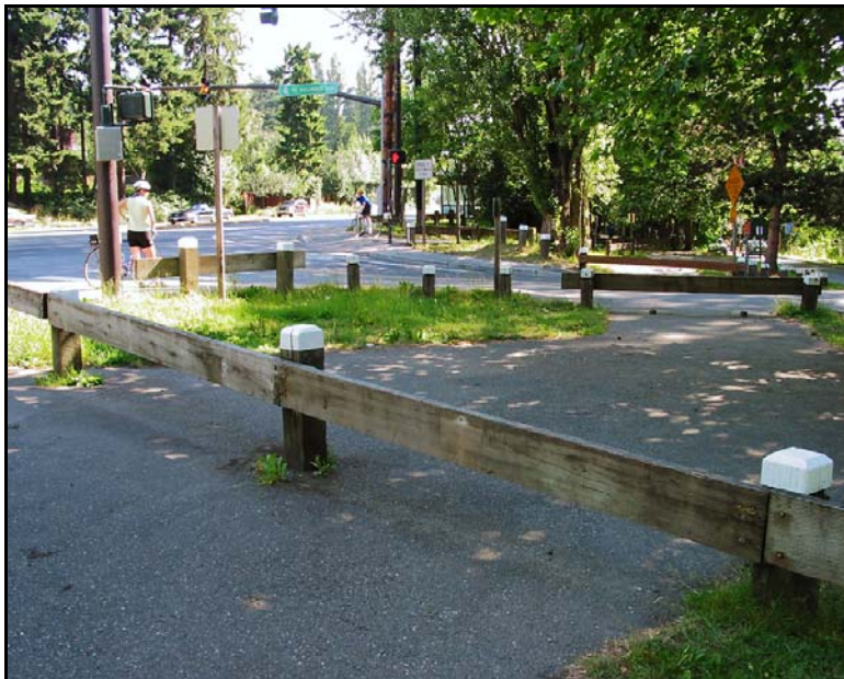
Figure 4.25 — Parallel pathway redirected to intersection
