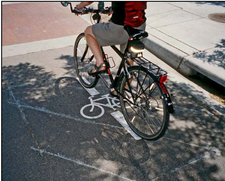
Figure 4.33 — Bicycle detector pavement marking
