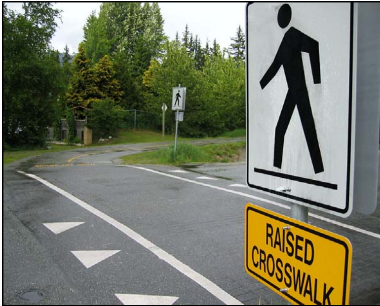
Figure 4.22 — Marked crossing with raised crosswalk
