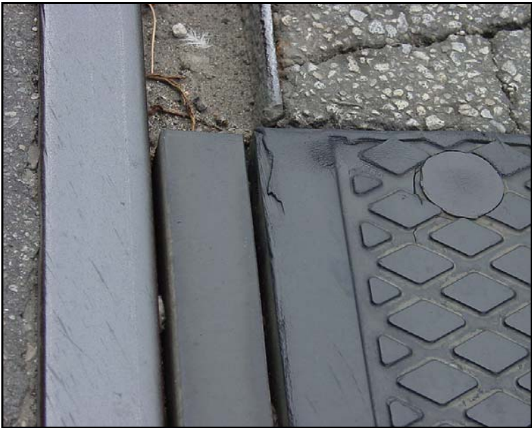
Figure 4.38 — Compressible flangeway filler
