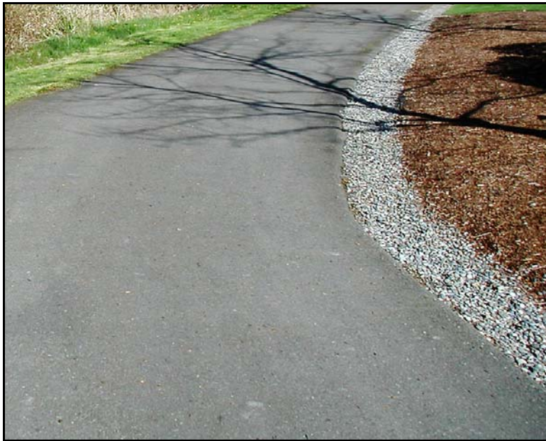
Figure 4.11 — Aggregate pathway shoulder
