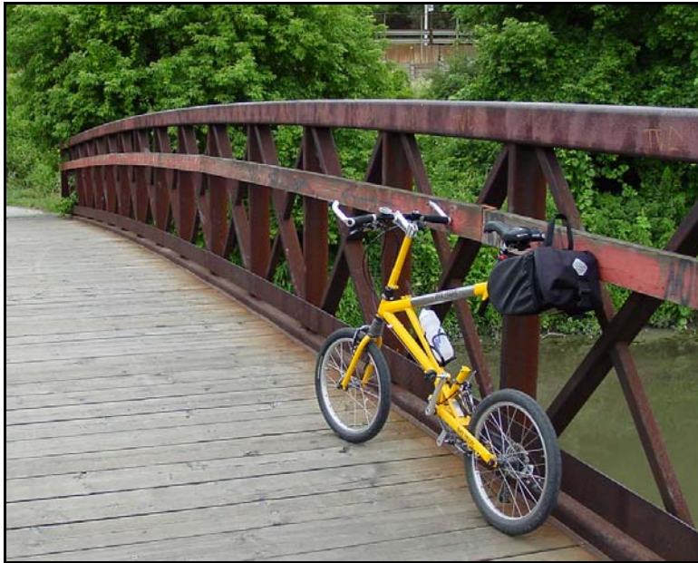
Figure 2.4 — Bridge on Pathway
