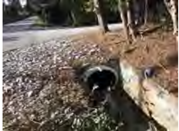
Photo A-46: Looking Downstream
