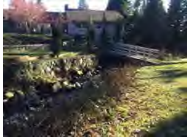
Photo A-114: Looking Downstream
