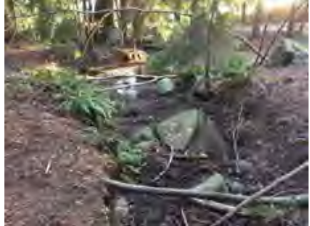
Photo A-150: Looking Downstream
