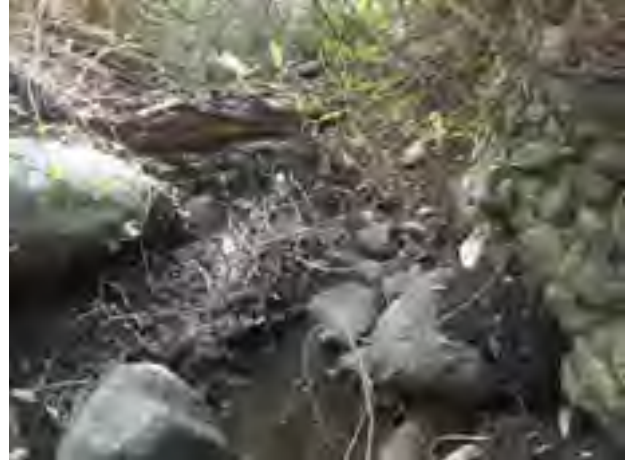
Photo A-138: Looking Downstream
