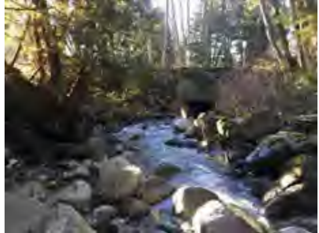
Photo A-34: Looking Downstream
