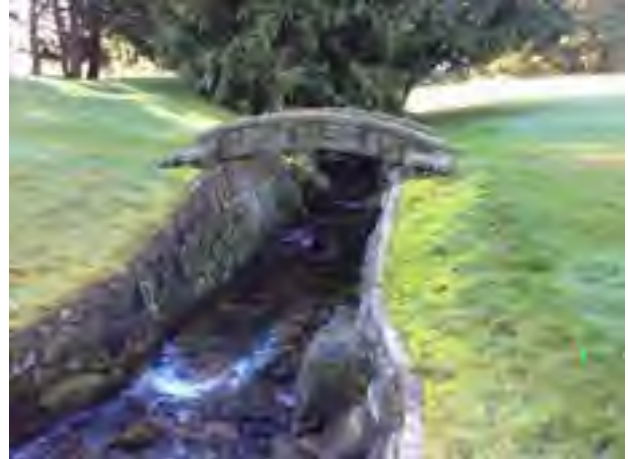
Photo A-106: Looking Downstream
