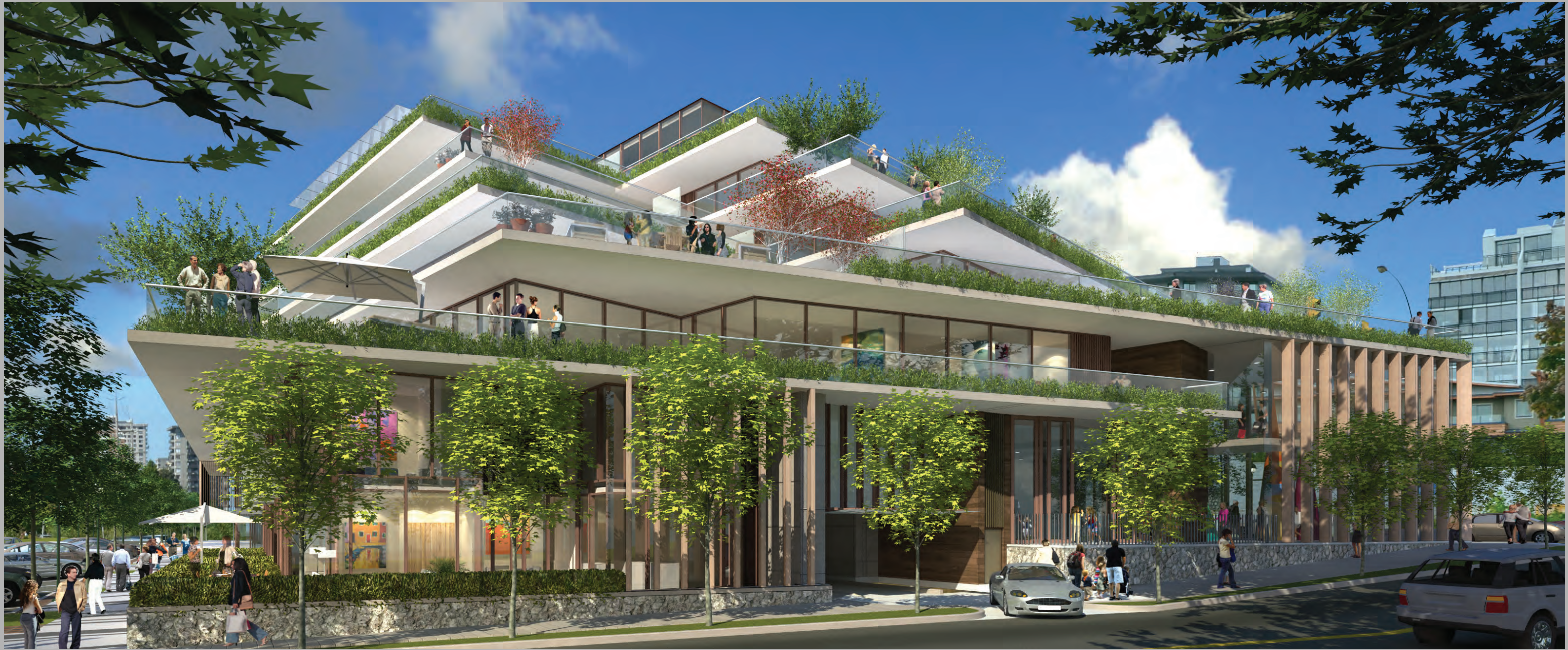
VIEW FROM CORNER OF 13TH STREET AND BELLEVUE AVENUE
