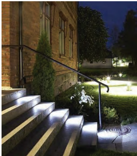
LED Orientation Luminaires_Erco
