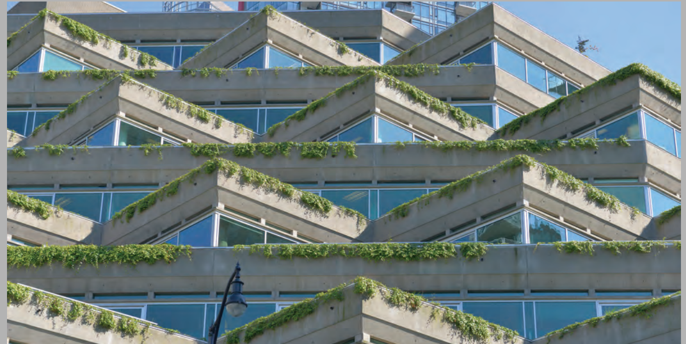
THE EVERGREEN BUILDING, ARTHUR ERICKSON, VICTORIA 1989
