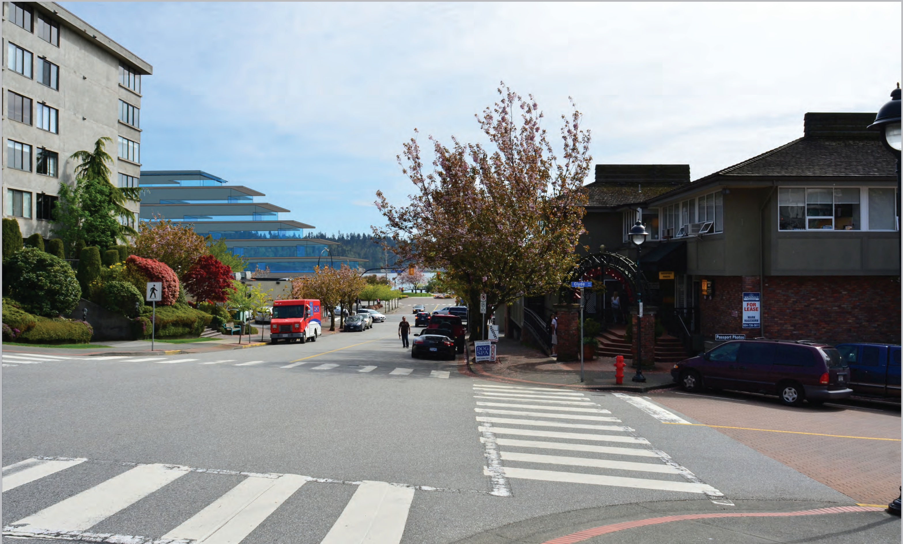
PUBLIC VIEW STUDY : VIEW FROM 14TH STREET AND CLYDE AVENUE ISSUED FOR CONCEPTUAL RESUBMISSION TO DRC - MAY 30, 2013
