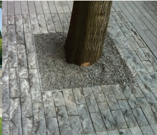
Crushed Gravel with Basalt Pavers
