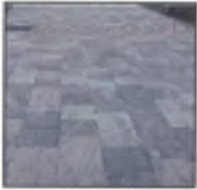
Rectangular Pavers at main walkways thru site
