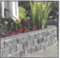
Low retaining wall around patios
