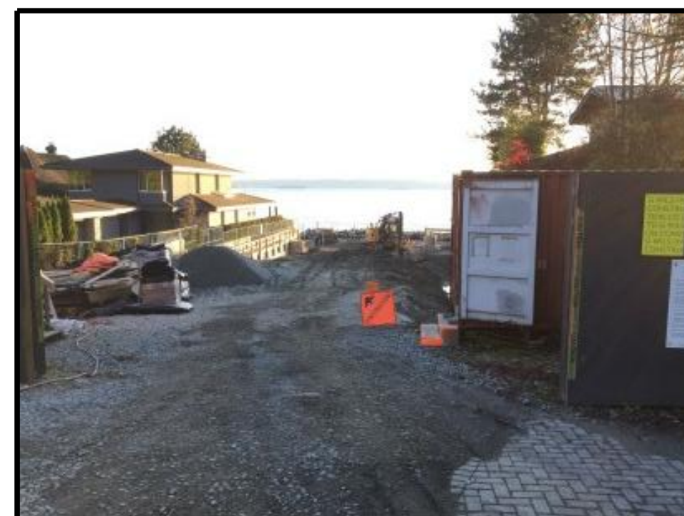
2882 Bellevue Avenue Year Built: Under Construction
