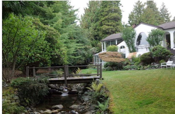
Photo 2. Looking upstream at Rodgers Creek and the existing bridge crossing and dwelling (2018-10-25).
