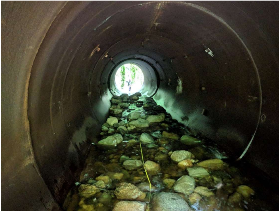
Figure 2. Rodgers Creek under railway, metal culvert – facing downstream (south)
