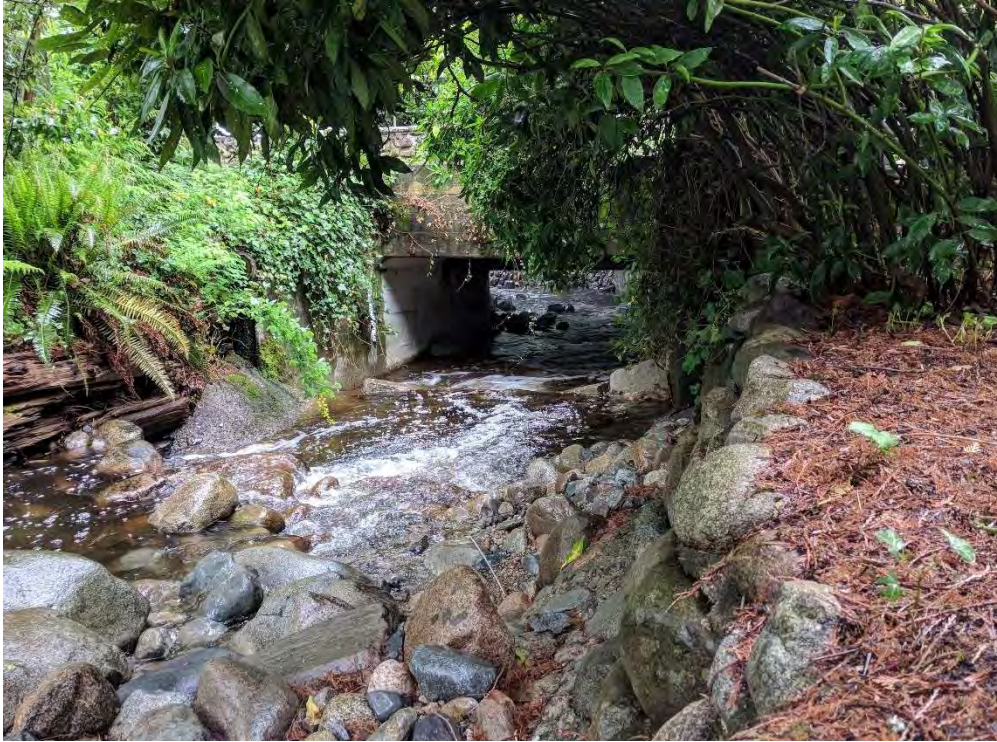
Figure 4. Rodgers Creek under Bellevue Ave, concrete culvert – facing downstream (south)
