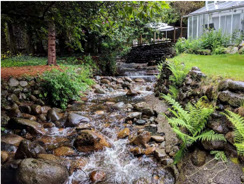
Figure 5. Rodgers Creek, concrete grouted cobble river wall along the covered swimming pool and typical channel section – facing upstream (northwest)
