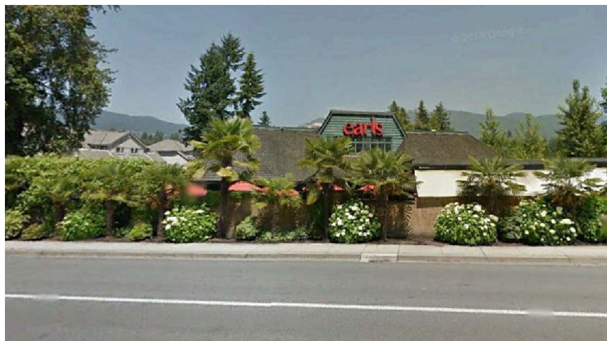
G SITE LOOKING NORTH
