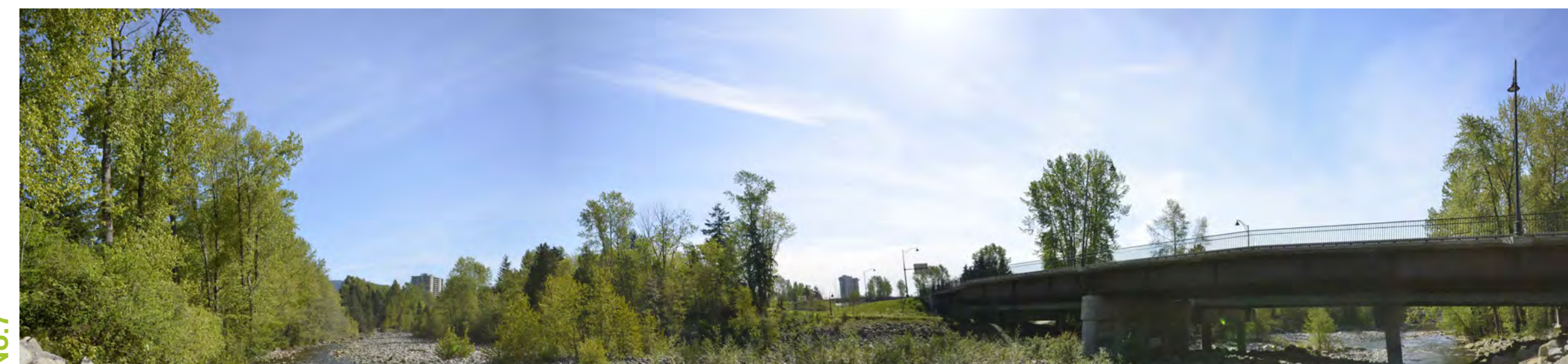
No.6 Taylor Way Looking East
