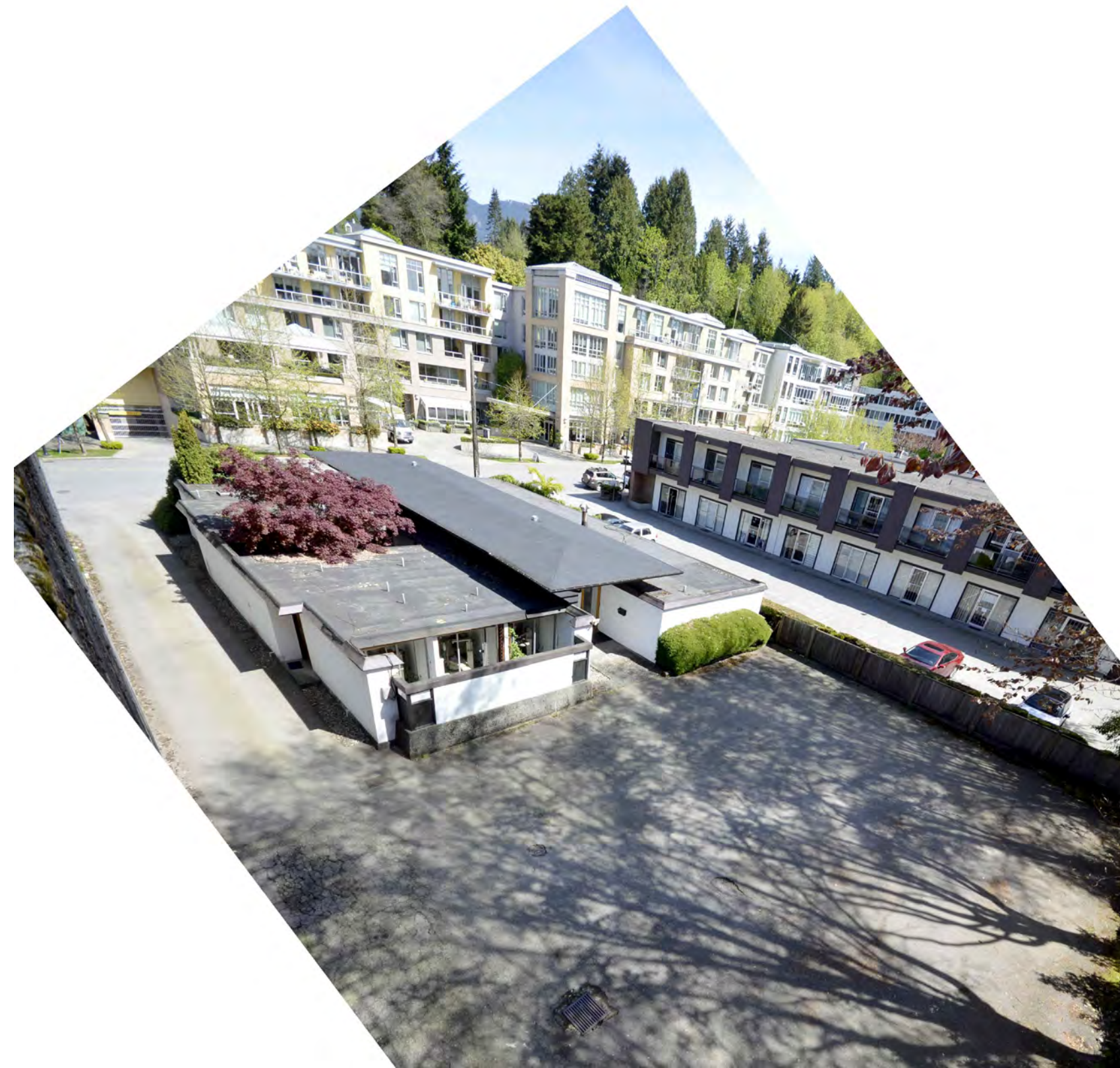
660 Clyde Avenue - Dental Clinic View Looking North
