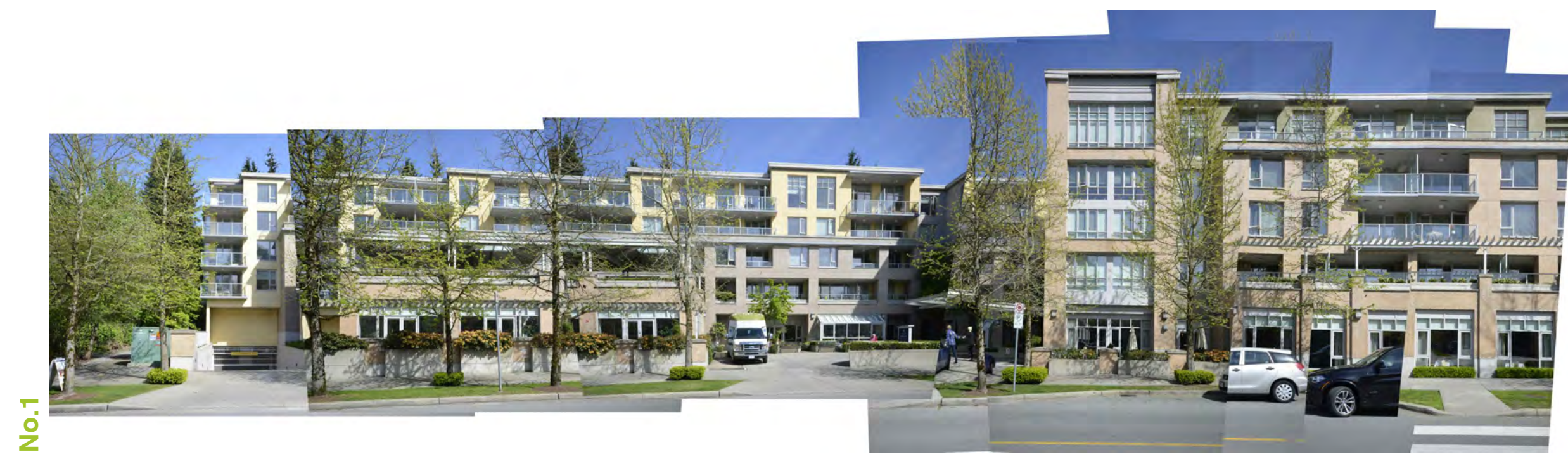
No.1 Clyde Avenue Looking North
