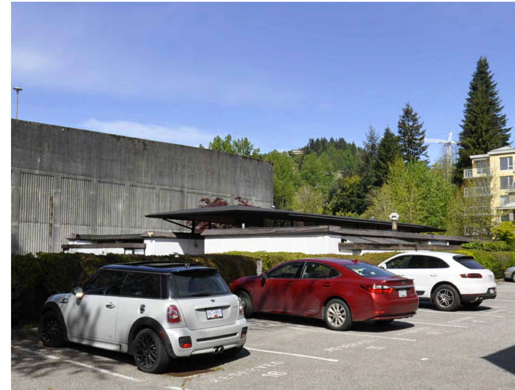
660 Clyde Avenue View from Adjacent Parking Lot
