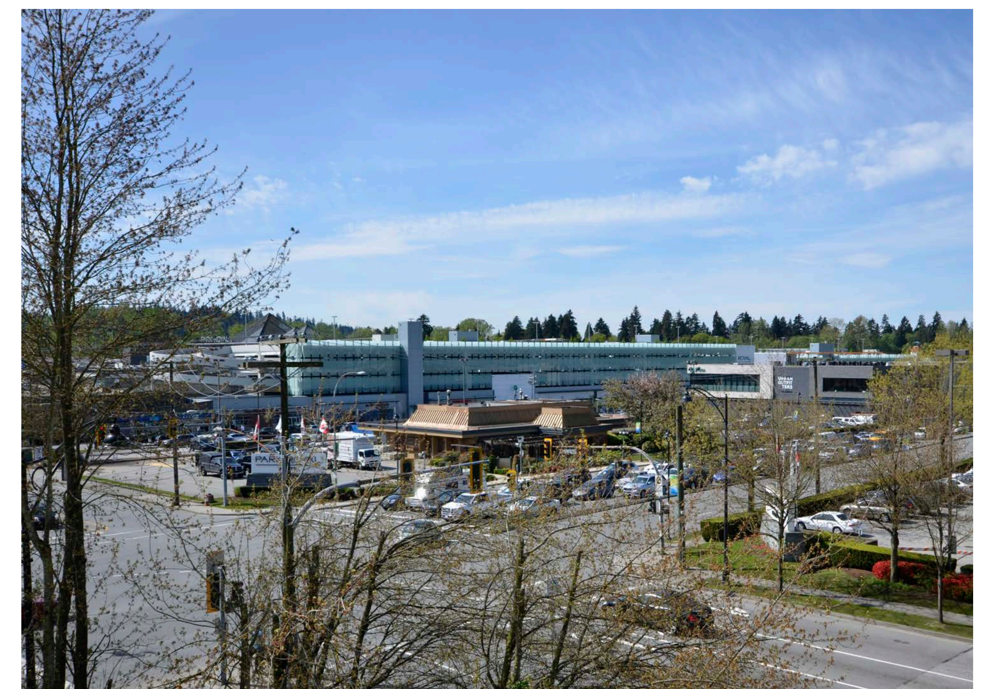
Park Royal Shopping Centre View Looking South East
