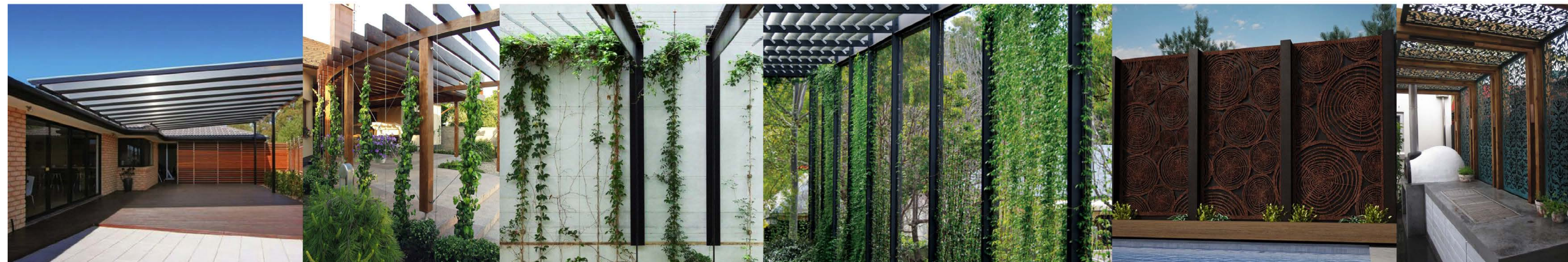
10 Metal beam pergola structures with water jet cut art panels and climbing vines in Mews L-5c NTS
