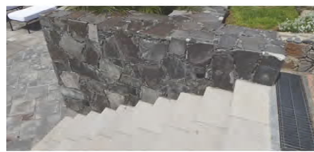
STONE WALL - FIN WALLS PROJECTING INTO LANDSCAPING
