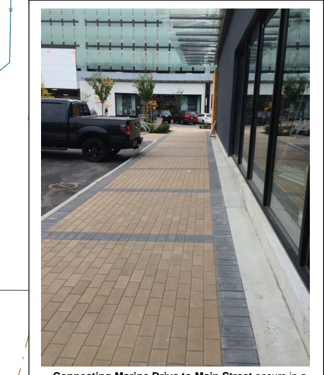
Connecting Marine Drive to Main Street occurs in a number of ways, but none more important than the open space adjacent to the Urban Outfitters. By opening up the space between the buildings and creating view and pedestrian corridors, we are connecting the spaces in a way that encourages pedestrians to explore the many spaces that Park Royal offers.
