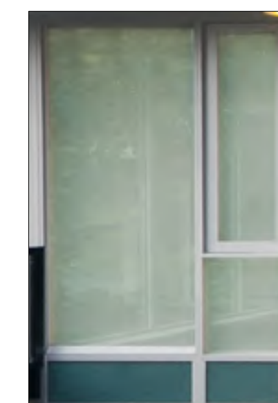
4 WINDOW WALL CLEAR GLASS PANEL, STANDARD SILVER FRAMES, AND "CLEAR GREEN" SPANDREL GLASS
