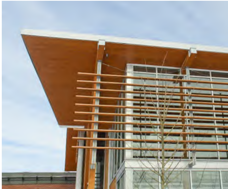
Solar shading devices, roof overhangs and balcony projections shelter high summer sun, but allow winter sun to penetrate
