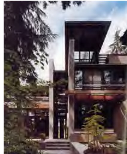
Architecture integrated into steep terrain
