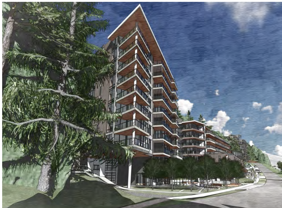
Solar shading devices, balcony projections and roof overhangs provide solar shading in summer, without excluding low-angle winter sun
