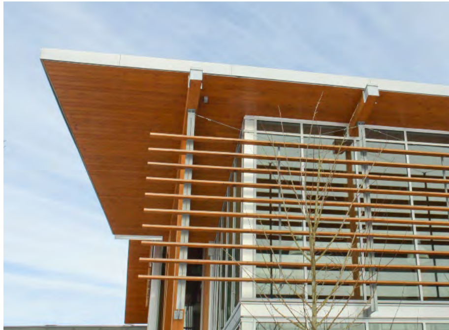
Solar shading devices, roof overhangs and balcony projections shelter high summer sun, while allowing winter sun to penetrate
