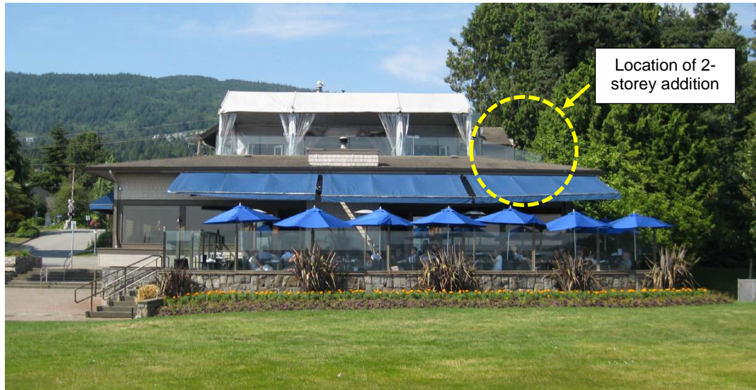
Figure 1: The Beach House Restaurant (before)
