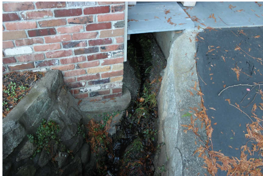
Photo 6. Outlet of concrete lined channel under existing deck. View looking upstream towards existing structure.
