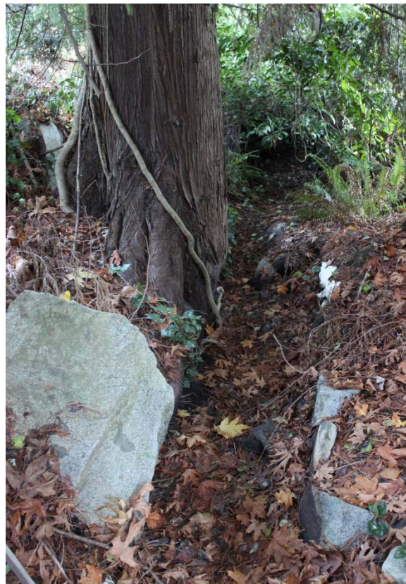
Photo 2. Manmade drainage channel running west to east along north boundary of property. View looking upstream (west).
