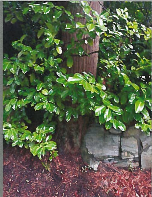
Photo 2: The existing rock wall is embedded into the trees trunk.
