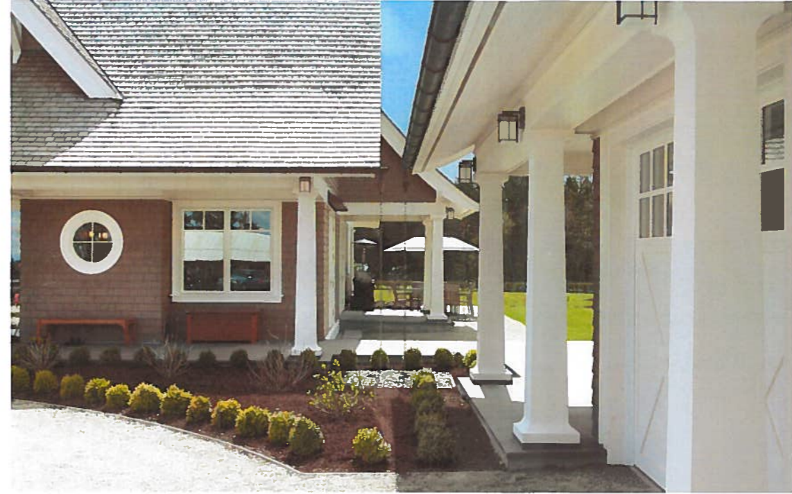
11 The materials, colours and textures of the exterior of the house will be reminiscent of the shingle-style craftsman houses built in West Vancouver a hundred years ago at the time lower Caulfeild was being developed. The columns, for example, will be in the rectangular form that carpenters built on site.
