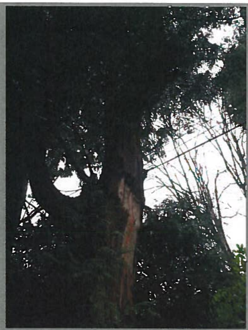
Photo 2: View of a previous replacement leader failure.
