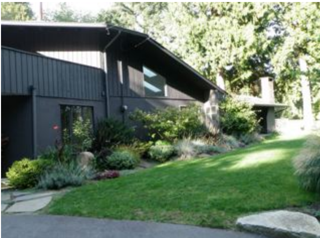
View of roof line to be removed, looking east
