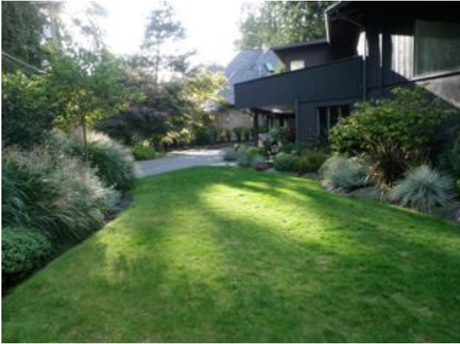
Front of dwelling; upper deck to be removed and new roof line established, looking west
