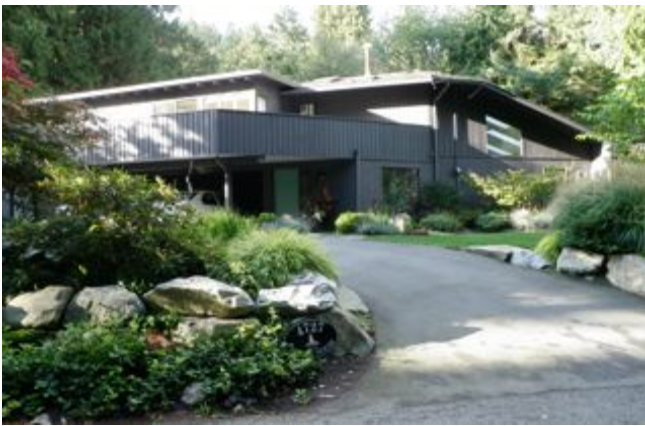
View from street, front deck to be removed
