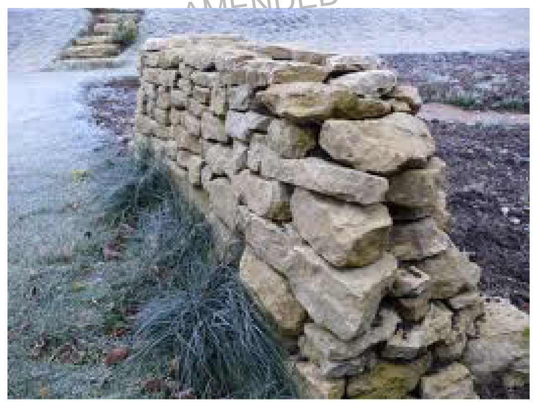
STONE WALL "RUIN"
