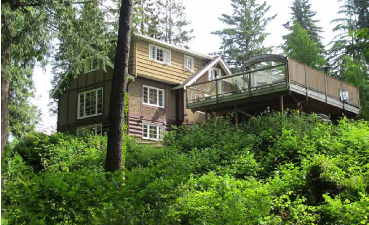
Below: West and rear elevation to the south, showing elevated porch beyond the surrounding native vegetation by the creek side.
