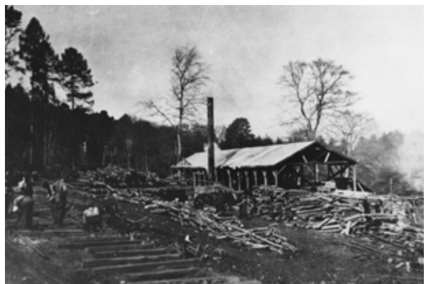
Robert Shields' Shingle Mill located at 15th street and Inglewood Avenue. Piles of wood and planks can be seen throughout the image along with men working, 1918, 1378.NSMA
