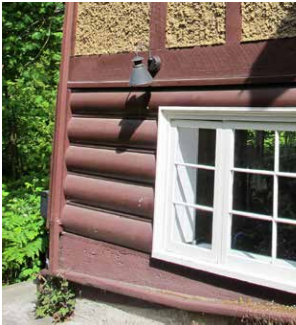
Typical condition of foundation, as seen from the southwest corner of the historic house.
