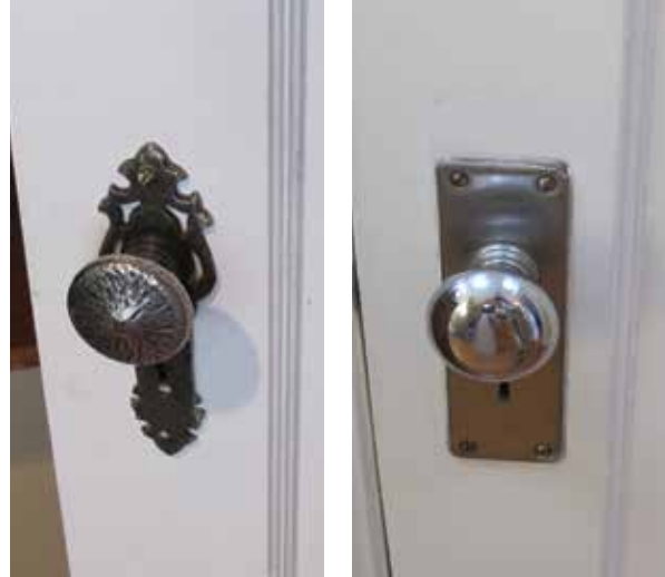
Existing metal door knobs of interior wooden doors.
