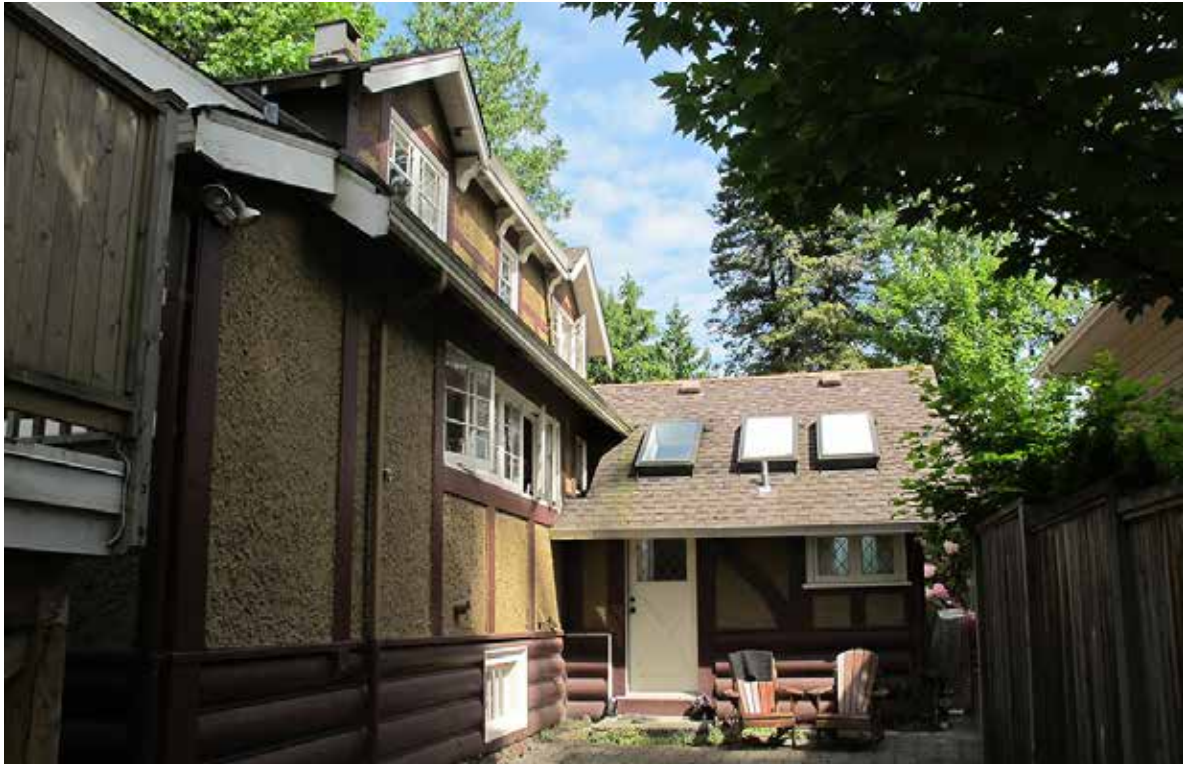
Partial east elevation and later side-gabled extension.
