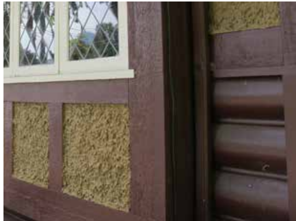
Photos showing typical condition of extant original wood trim work of the historic house, as seen from the ground.
