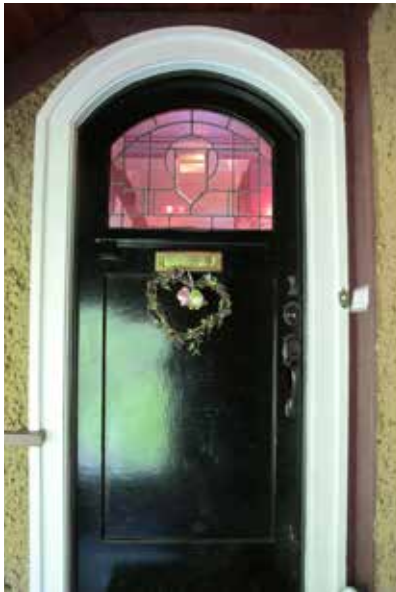
Photos showing existing exterior wood doors in different configurations and locations: the original wooden front door at the west return of the front facade to the north (left); and south elevation (right). Note that all doors feature multi-pane leaded glass windows and true-divided lights.
