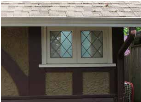
Photos showing typical condition of extant exterior wood windows in different configurations.
