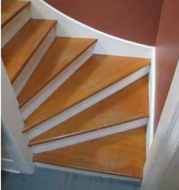
Photos showing newel post (top) and configuration of main staircase with winders (bottom).
