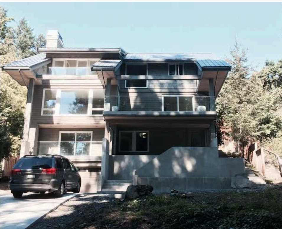
Neighboring homes on Piccadilly South. The new home has been designed to have a similar appearance of existing homes on Piccadilly South.
