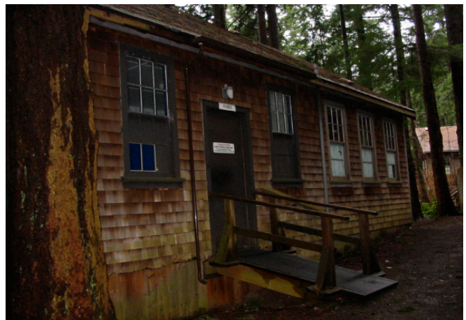
Top: Concrete steps and railing Centre: Stone retaining wal Bottom: Wooden barracks
