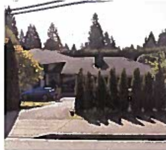
2 740 Inglewood Ave looking south
