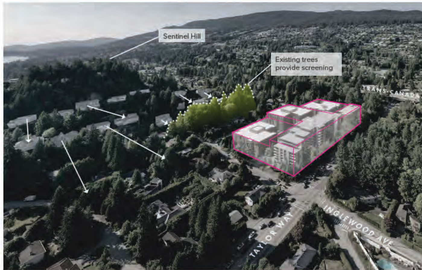
A Aerial view looking North West
