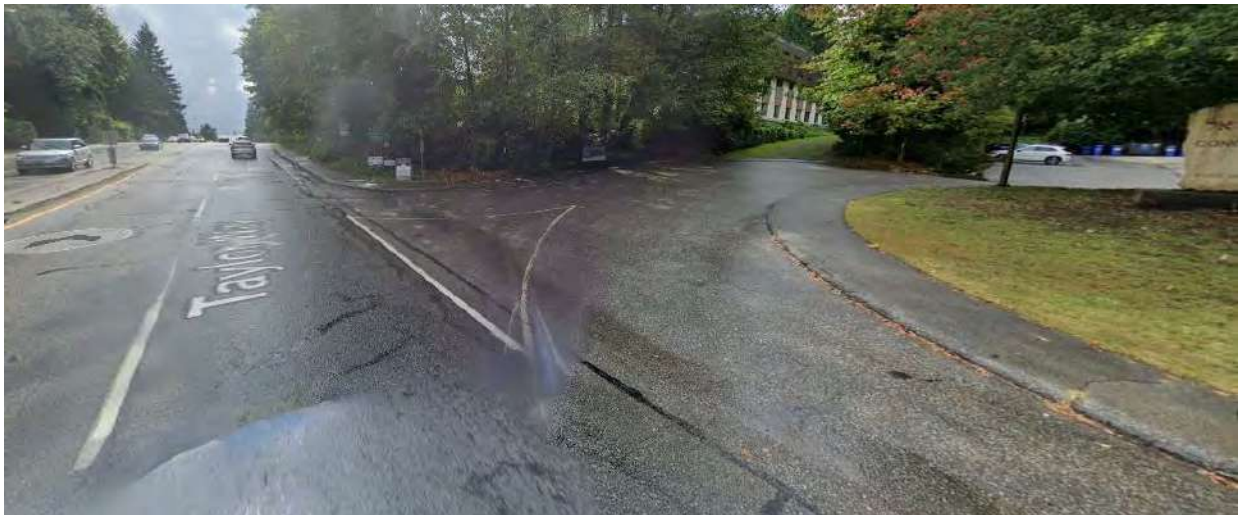
Figure 2.1: Existing Taylor Way Access Looking Southbound
