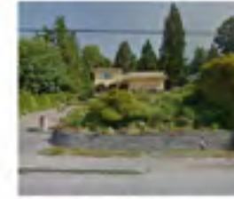
PHOTO 03: EXISTING DWELLING (707 KEITH ROAD)
