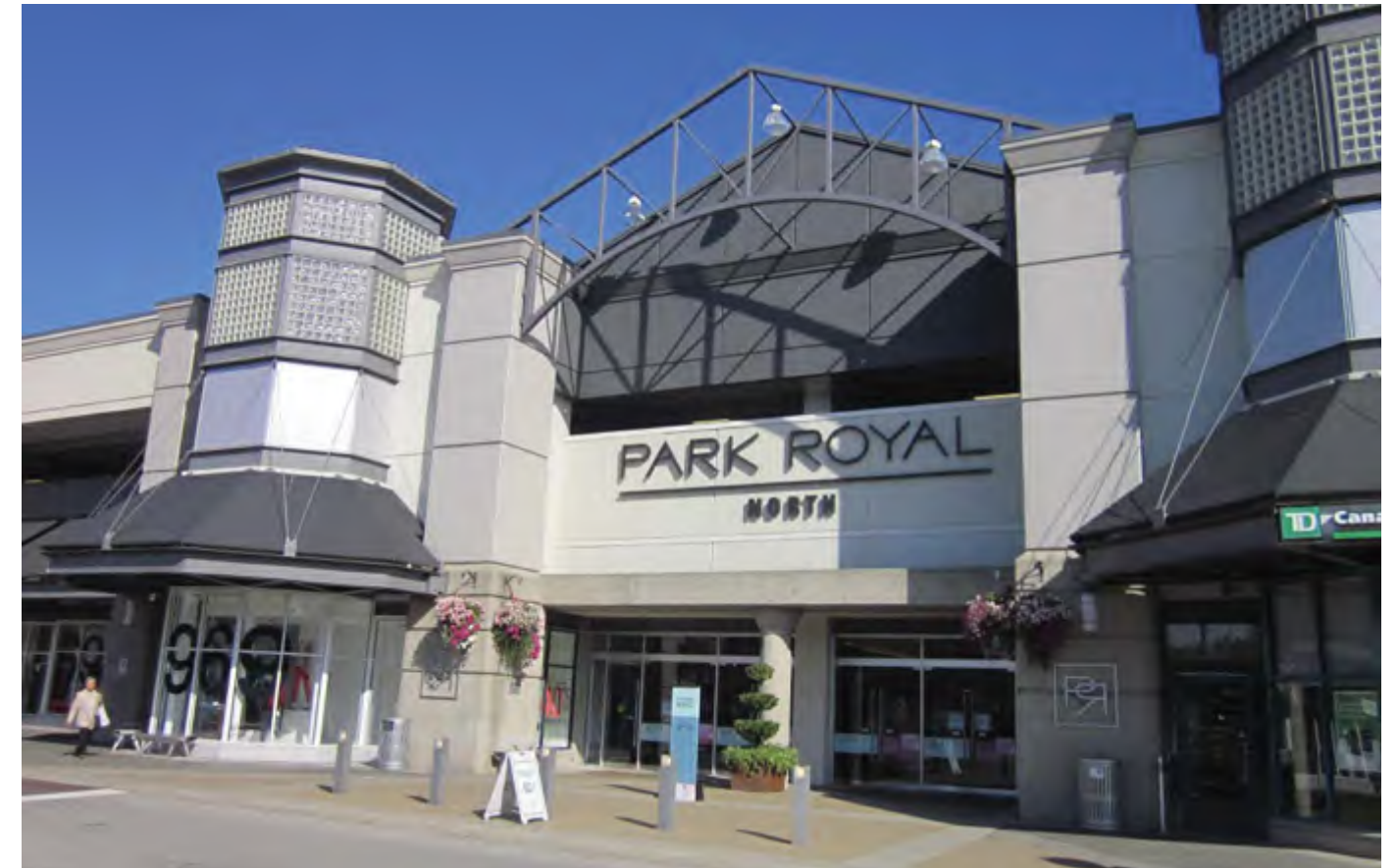
EXISTING FACADE TREATMENT
