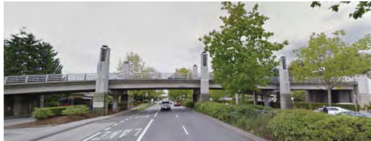
EXISTING OVERPASS ROAD FALSE COLUMNS
