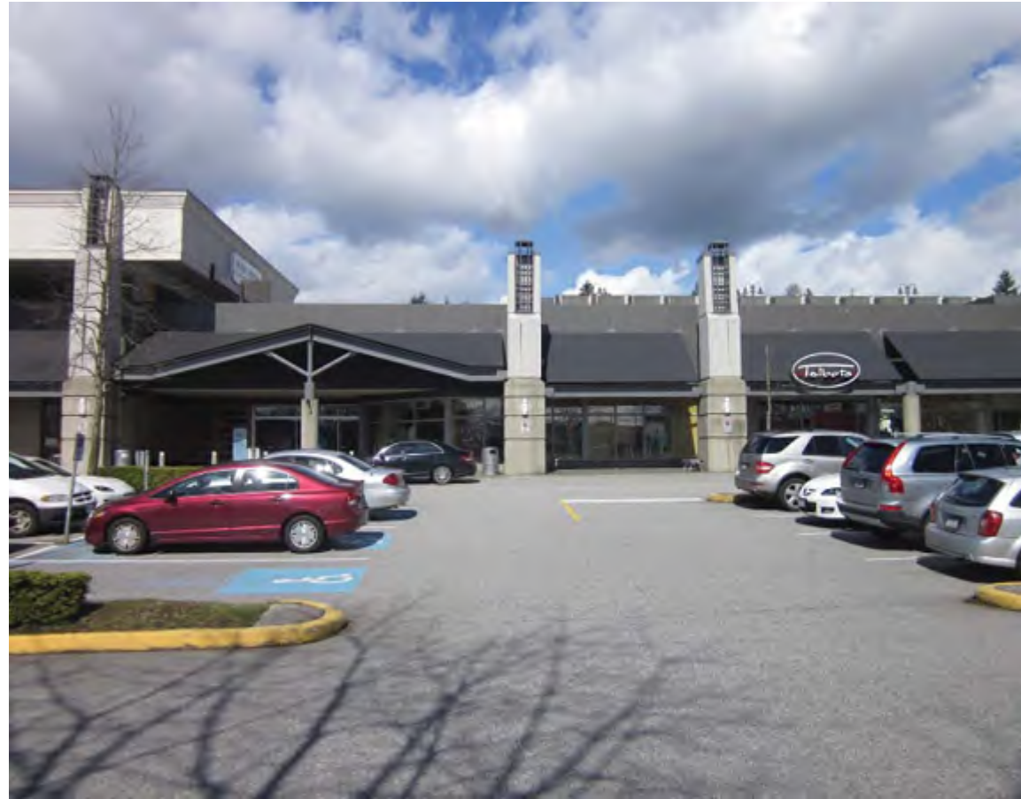
PARK ROYAL NORTH MALL SECONDARY ENTRANCE - EXISTING
