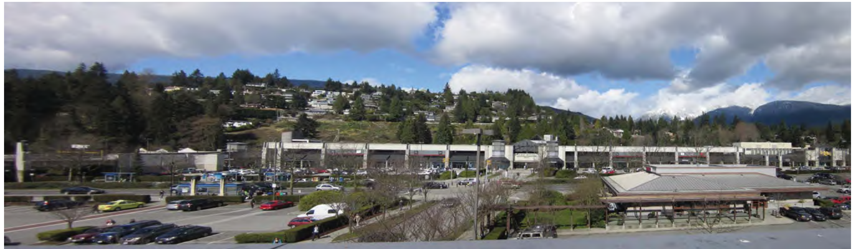
PARK ROYAL NORTH - EXISTING VIEW FORM THE PARKADE ROOF OF BUILDINGS B&C
