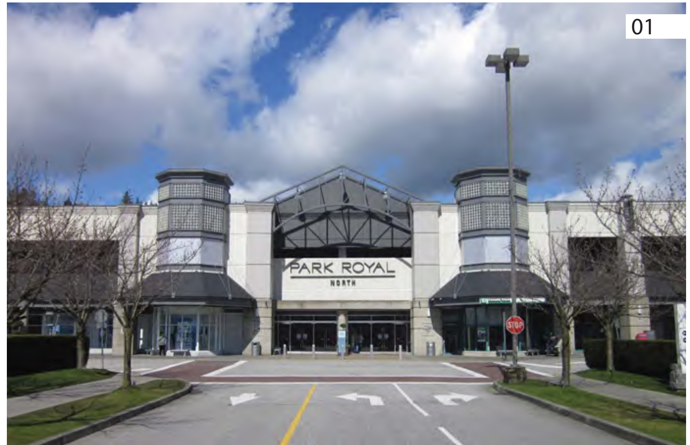
EXISTING PARK ROYAL NORTH MALL MAIN ENTRANCE
