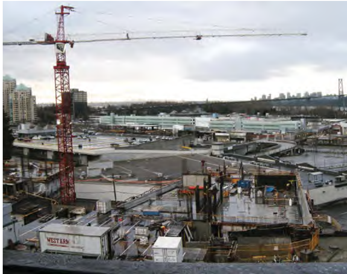
VIEW FROM EVELYN DRIVE DEVELOPMENT - EXISTING
