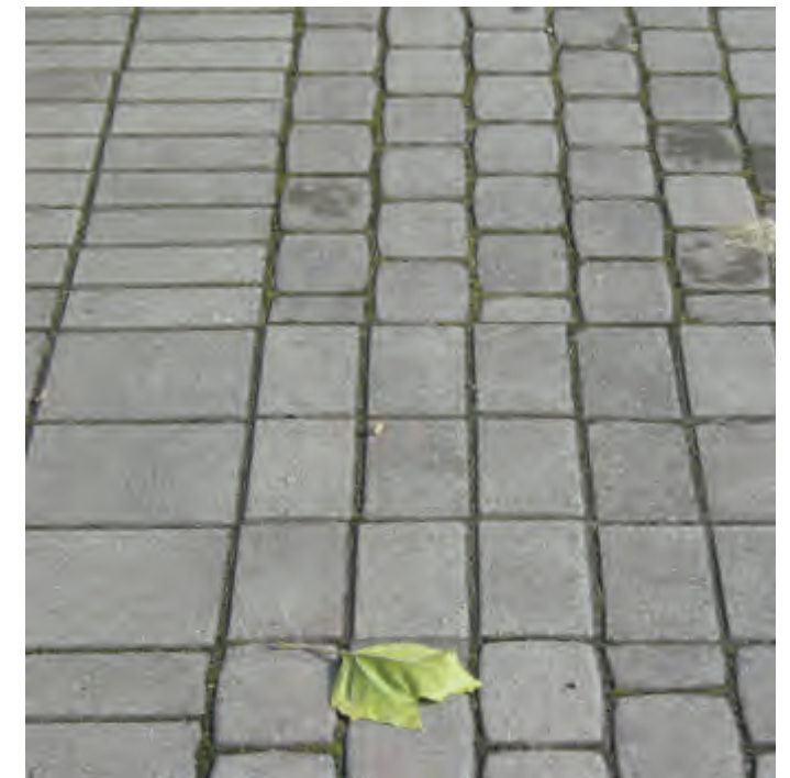
Permeable paving helps with stormwater management
