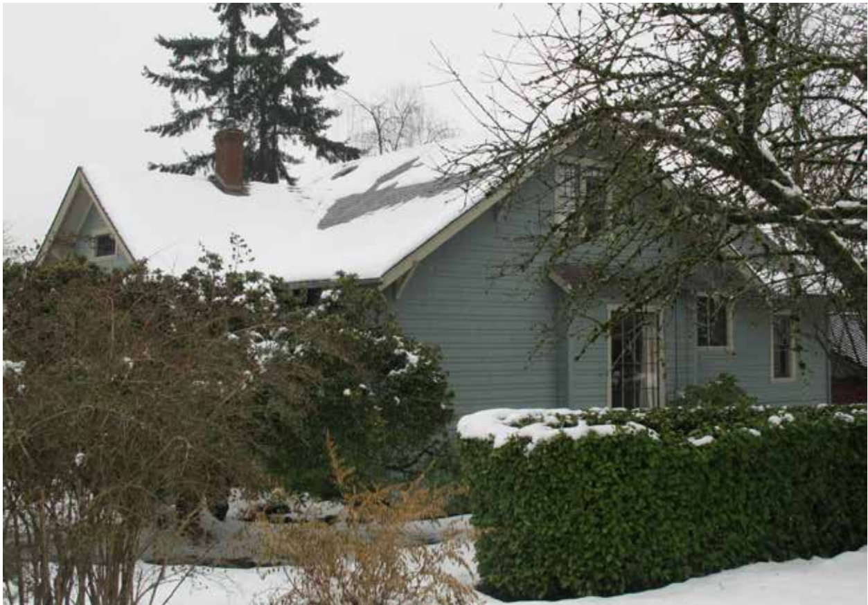
side elevation of the Rush House, at corner of 12th Street and Jefferson Avenue.
