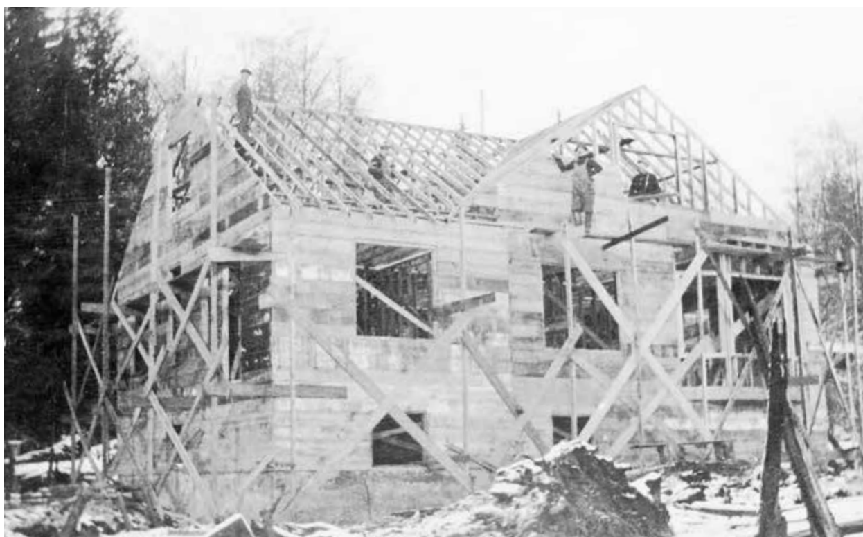
Rush House under construction, 1923. (3267.WVA.PHO)
