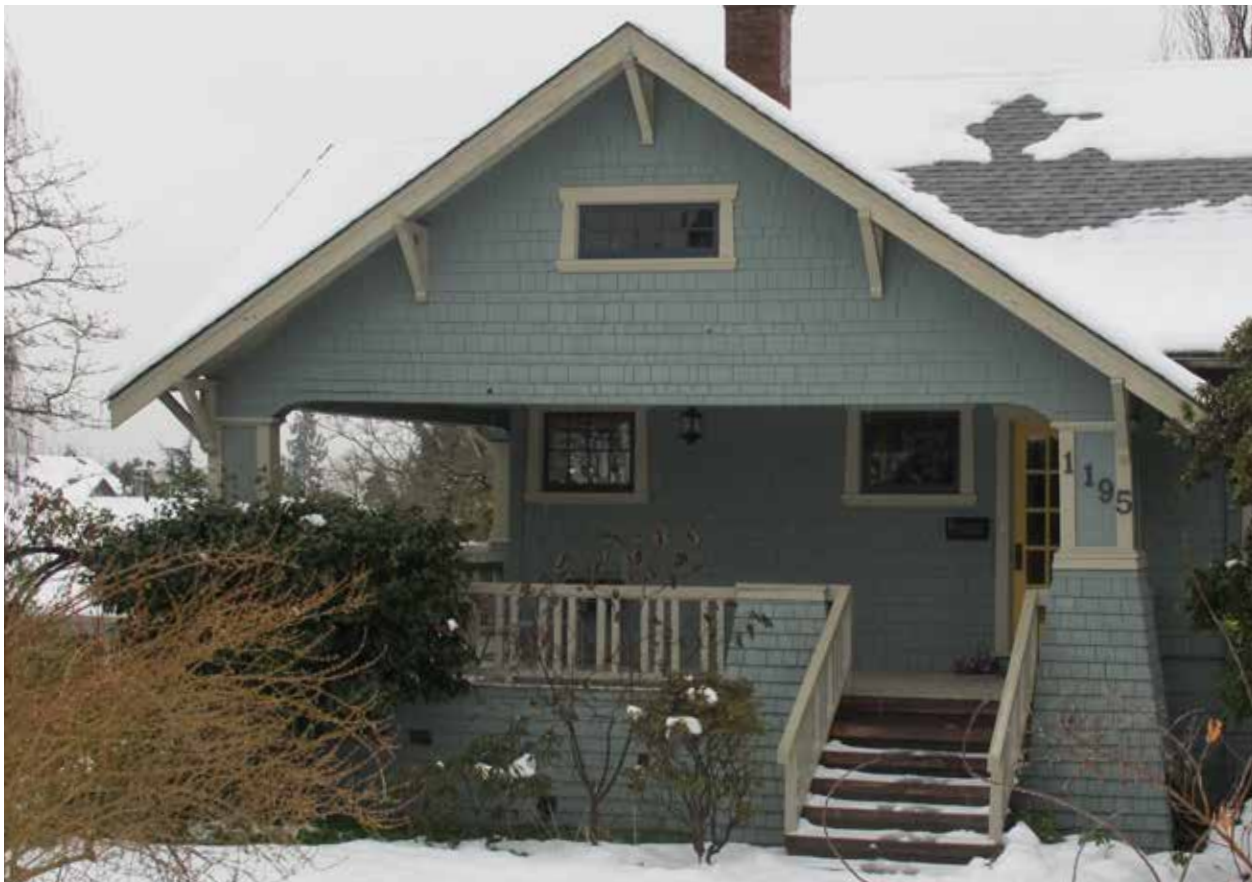
Wrap-around verandah of the Rush House, facing 12th Street.
