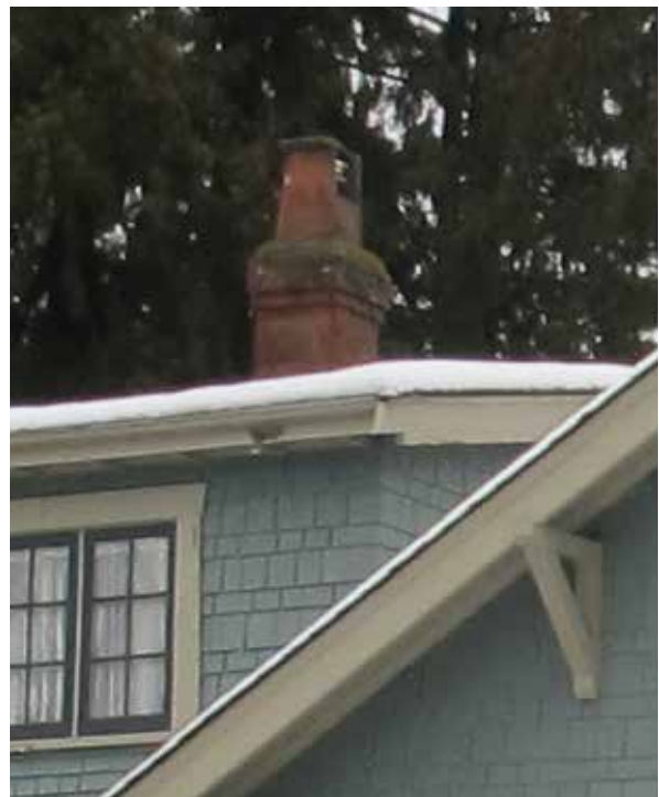
Interior brick chimneys of the Rush House.
