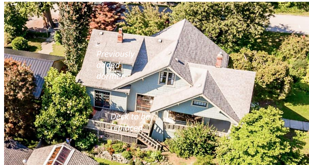
The 1970s deck along the south side of the house will be removed along with the French doors and large windows and replace with more traditional windows.
