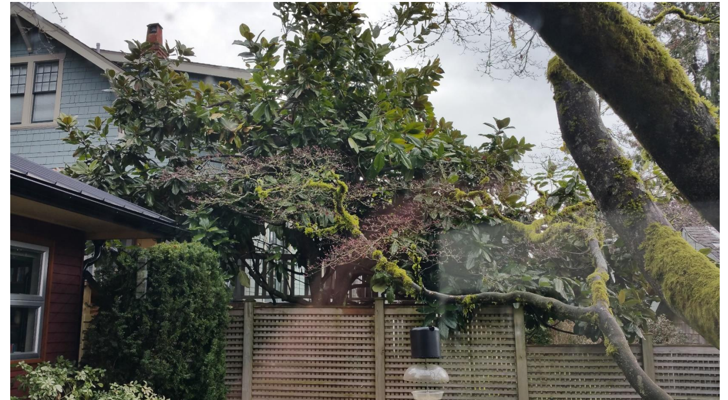
View of Rush House as seen from the kitchen/family room of the house to the west
