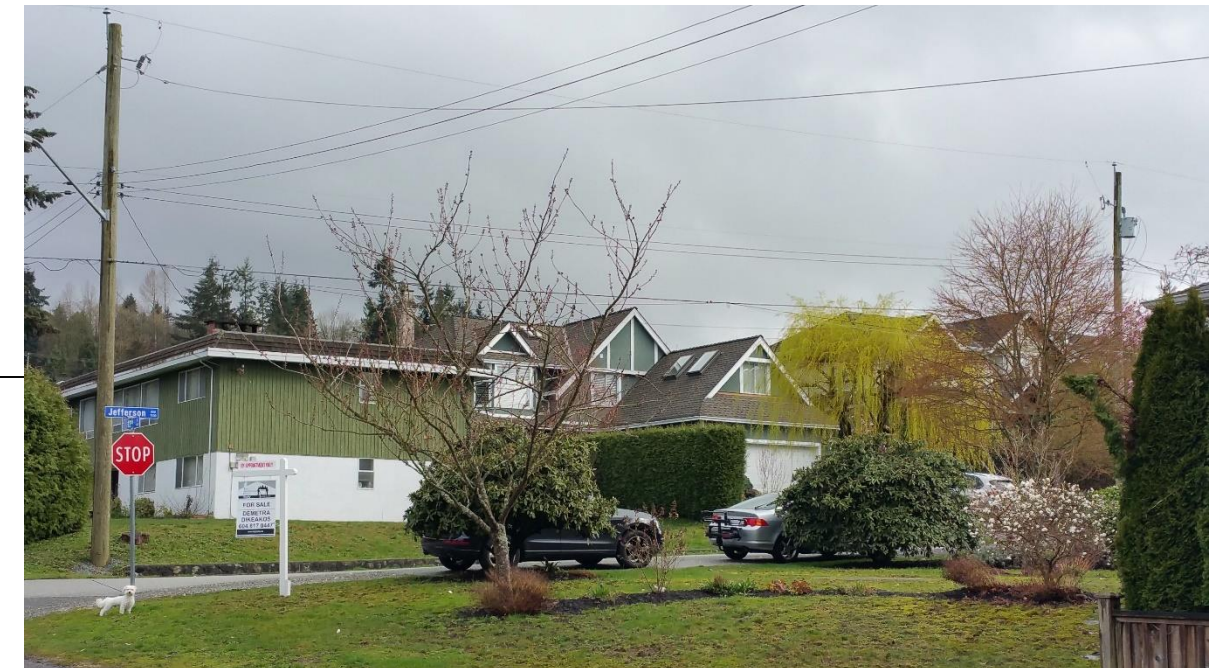
View of house to north-east at corner of Jefferson Avenue and 12 th Street
