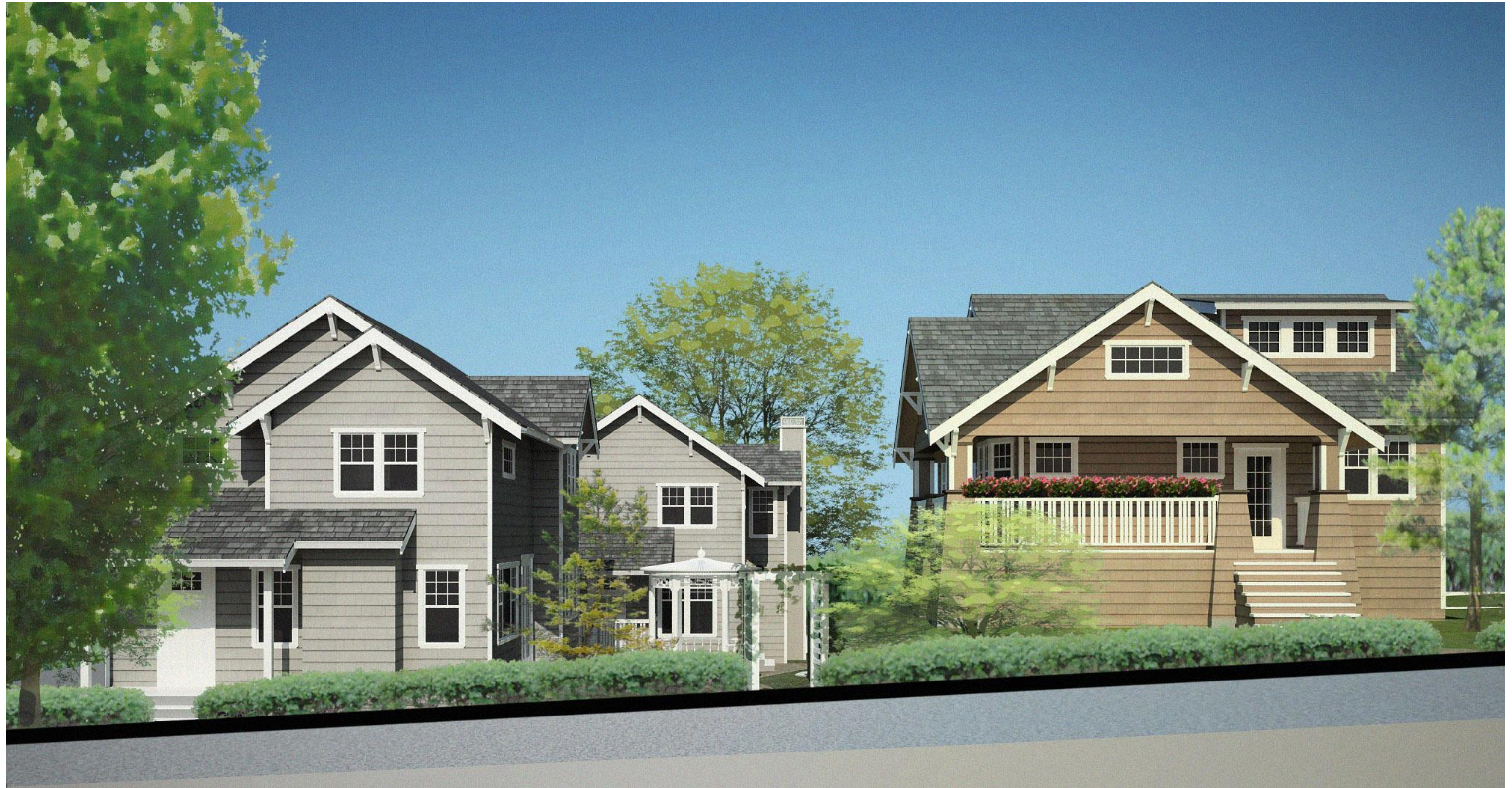
The view along 12 th Street illustrating the earlier proposal to use the same colour for the Laneway and Garden Cottages. However, as a result of the Design Review Committee recommendations, different but complementary heritage colours are now proposed for the two infill cottages, along with a mix of shingles and horizontal siding similar to the existing Rush House
