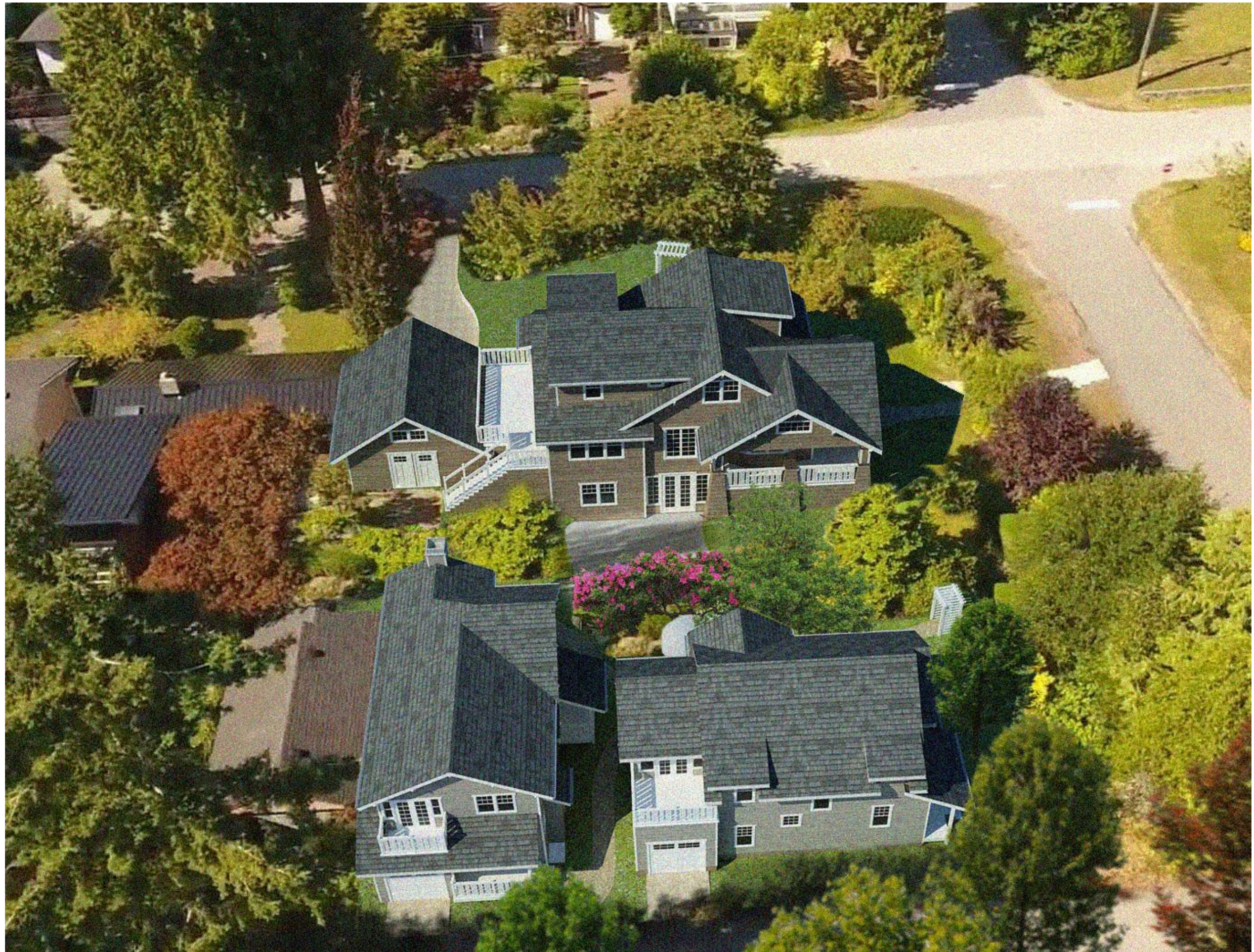
An earlier Bird's eye view looking north (Note: the rear deck between Rush House and the garage structure has subsequently been revised in response to the DRC comments)
