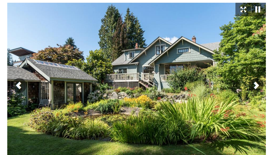
While alterations have been made to the house over the years, it is in good condition and lends itself to conservation and renovation and a return to its former significance and glory.
