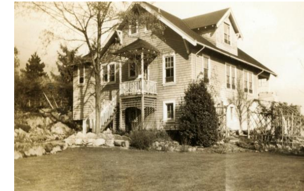
Kilby house 1930's
