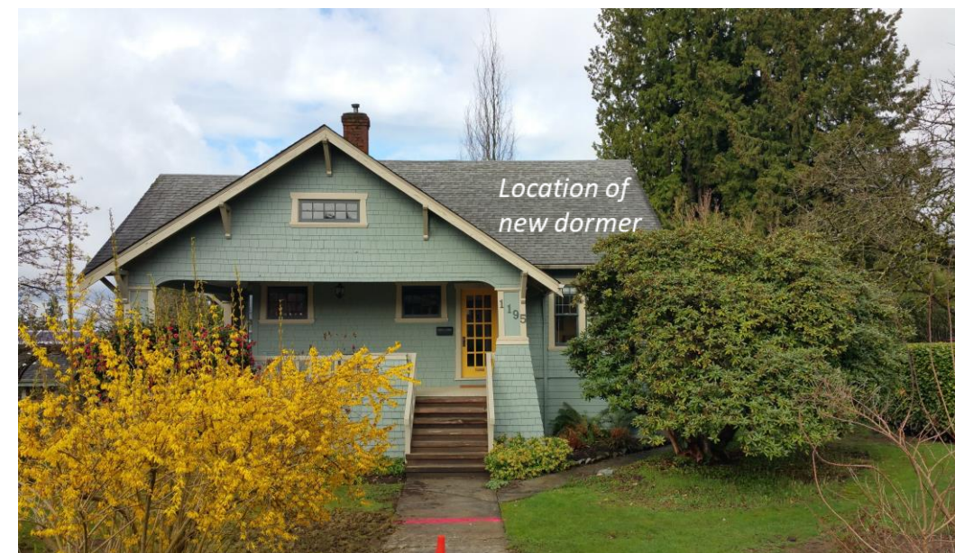
A new dormer is proposed for the 12th Street façade, similar to the dormer that was added along the south façade (see middle photo)
