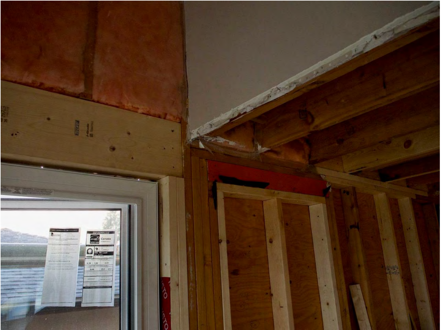
This picture is a closet shot of the attic floor joist over second floor wall plate
