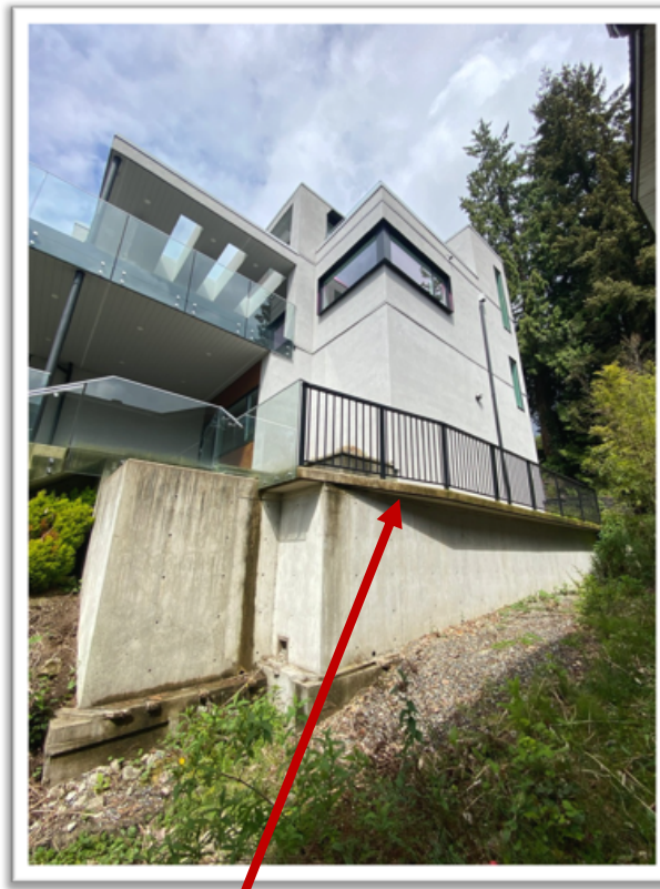
The proposed Lower Floor Elevation will be 14 feet lower than neighbor's basement elevation.
