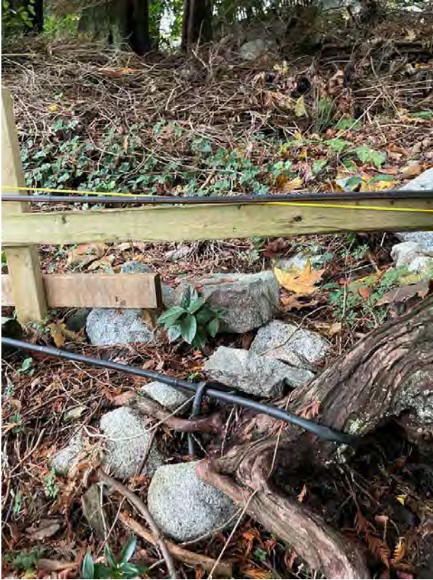
Figure 1: Fallen Rock Debris
