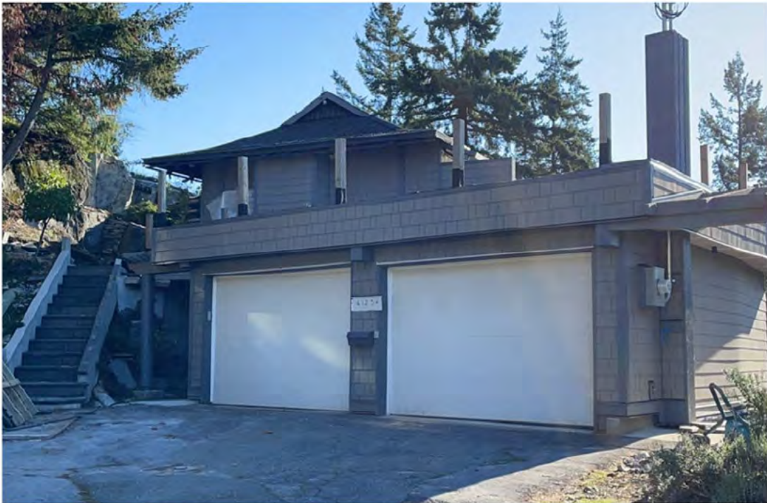
Now (Garage extension has been constructed)
