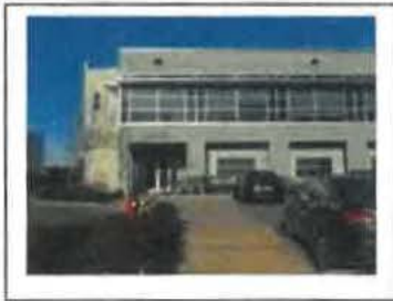
Pedestrian access from street to front entrance of building
