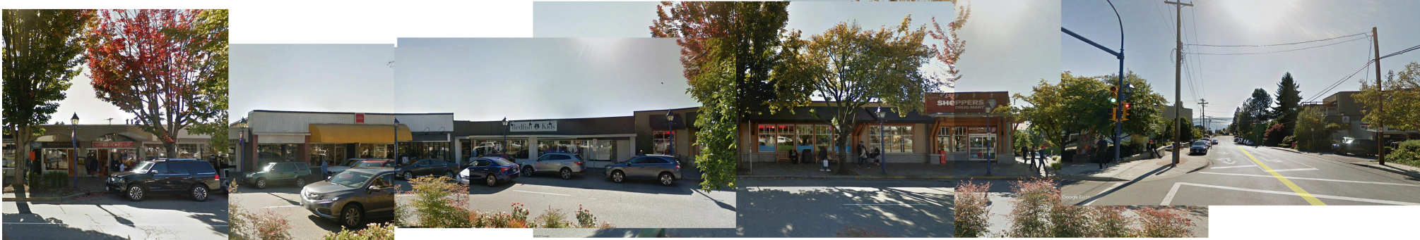
3. MARINE DRIVE (SOUTH) - FACING SITE
