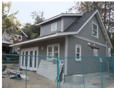
Level ‘B’ Coach House (nearing completion)
