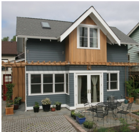
Backyard Cottage, Seattle
