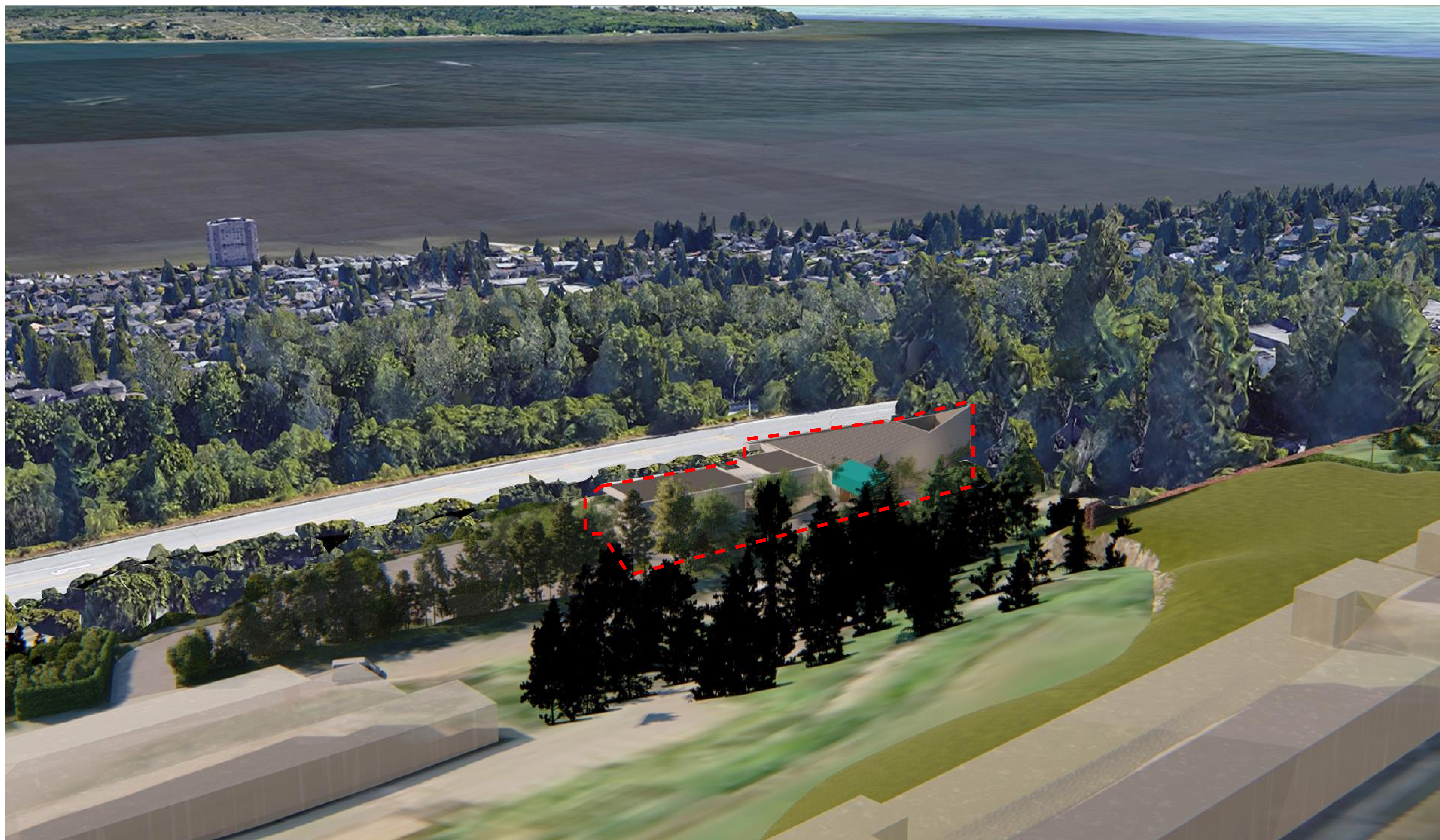
EXISTING SOUTH WEST VIEW
