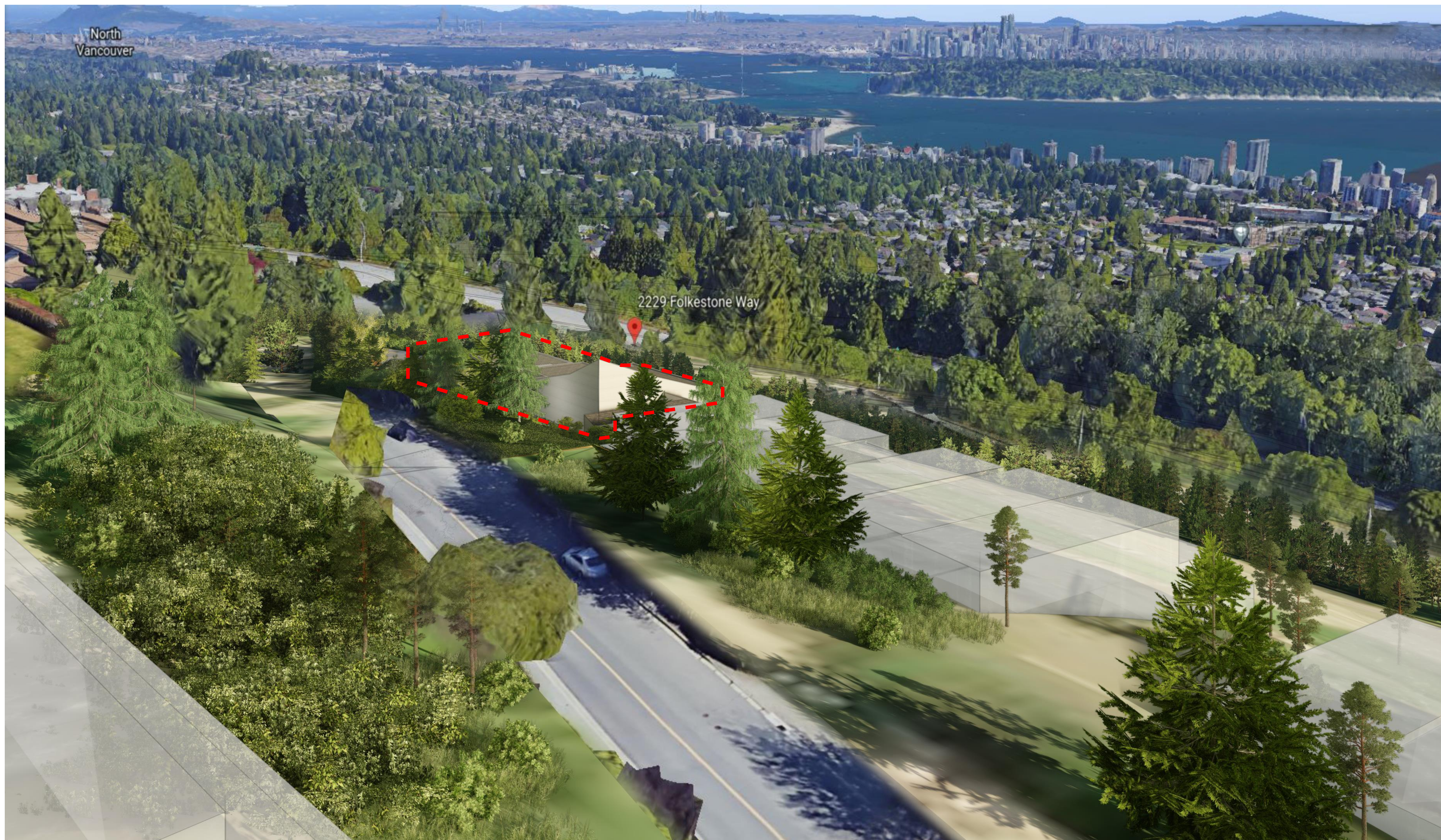
EXISTING SOUTH EAST VIEW
