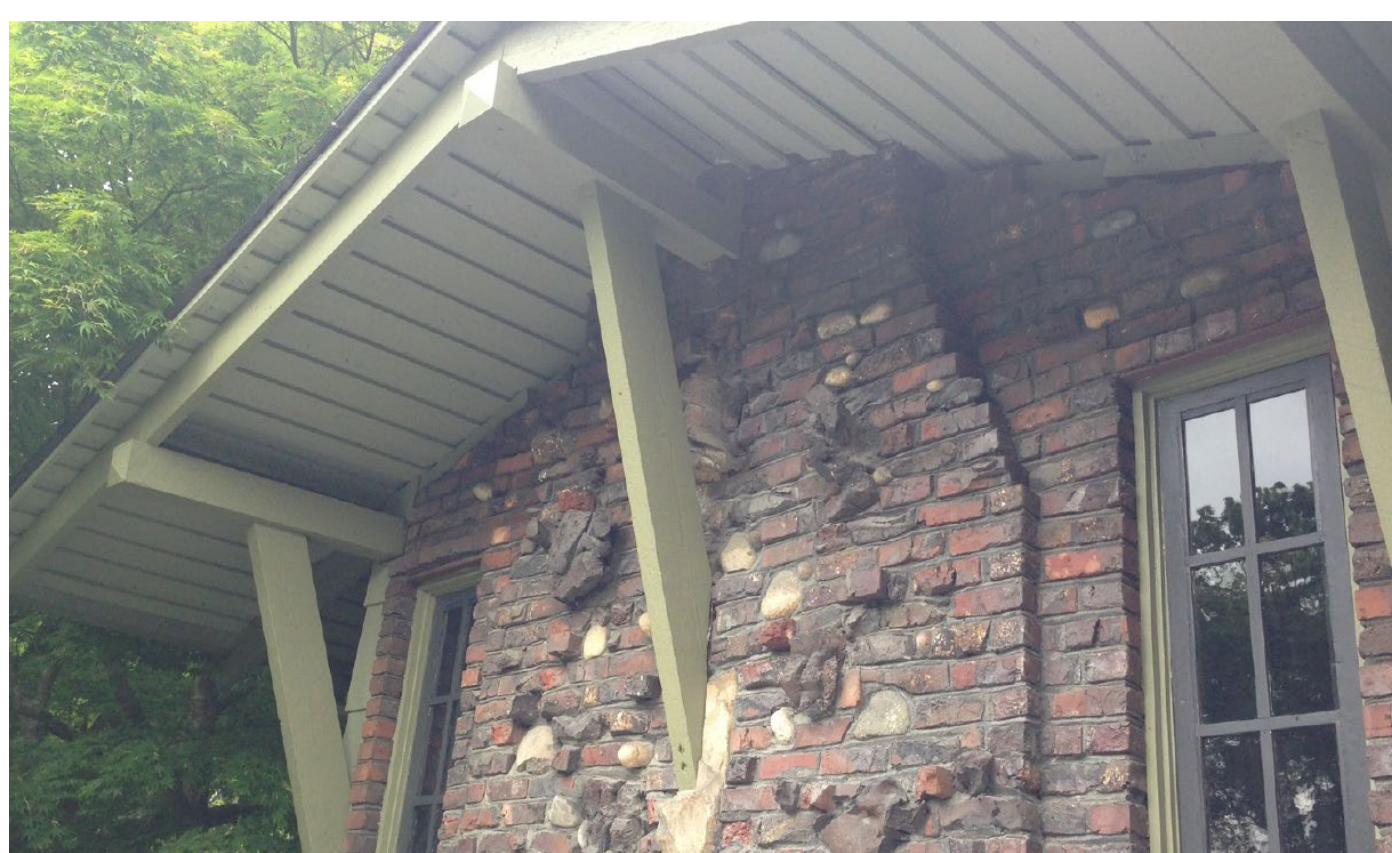
The Doctor-Stewart heritage house is notable for its extensive use of clinker brick and river rock, as featured in this massive fireplace.
