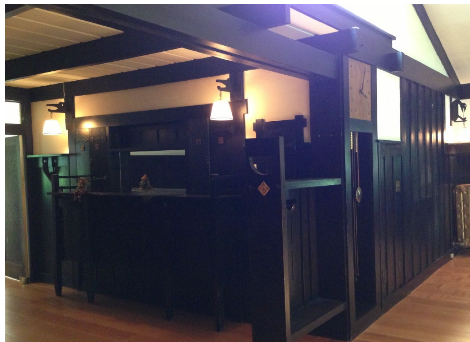
Dining room with original plywood salmon and bird lights, built in long-case clock, built-in sideboard, hand-made tiles, and pressed-steel radiators.
