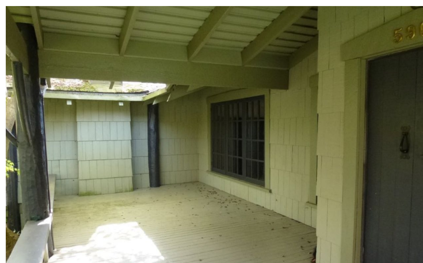
Arts & Crafts homes, including the Doctor-Stewart house, were constructed using local materials and traditions, including these adzed log pillars, hand-hewn fir door, exposed rafters, and extra long shingles.
