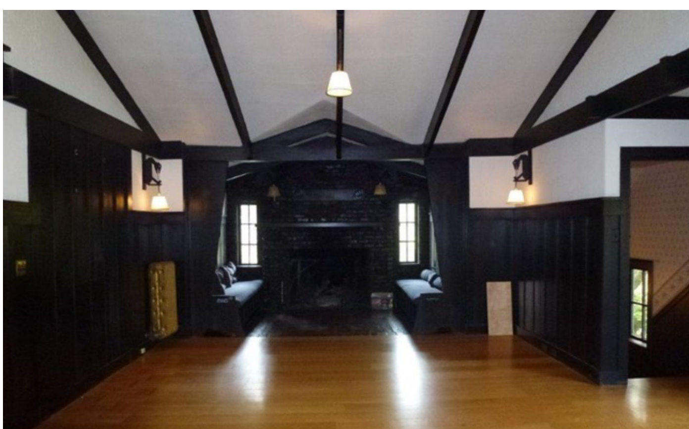
The living room inglenook featuring unique plywood bird lights, pressed-steel radiators, and clinker-brick fireplace.
