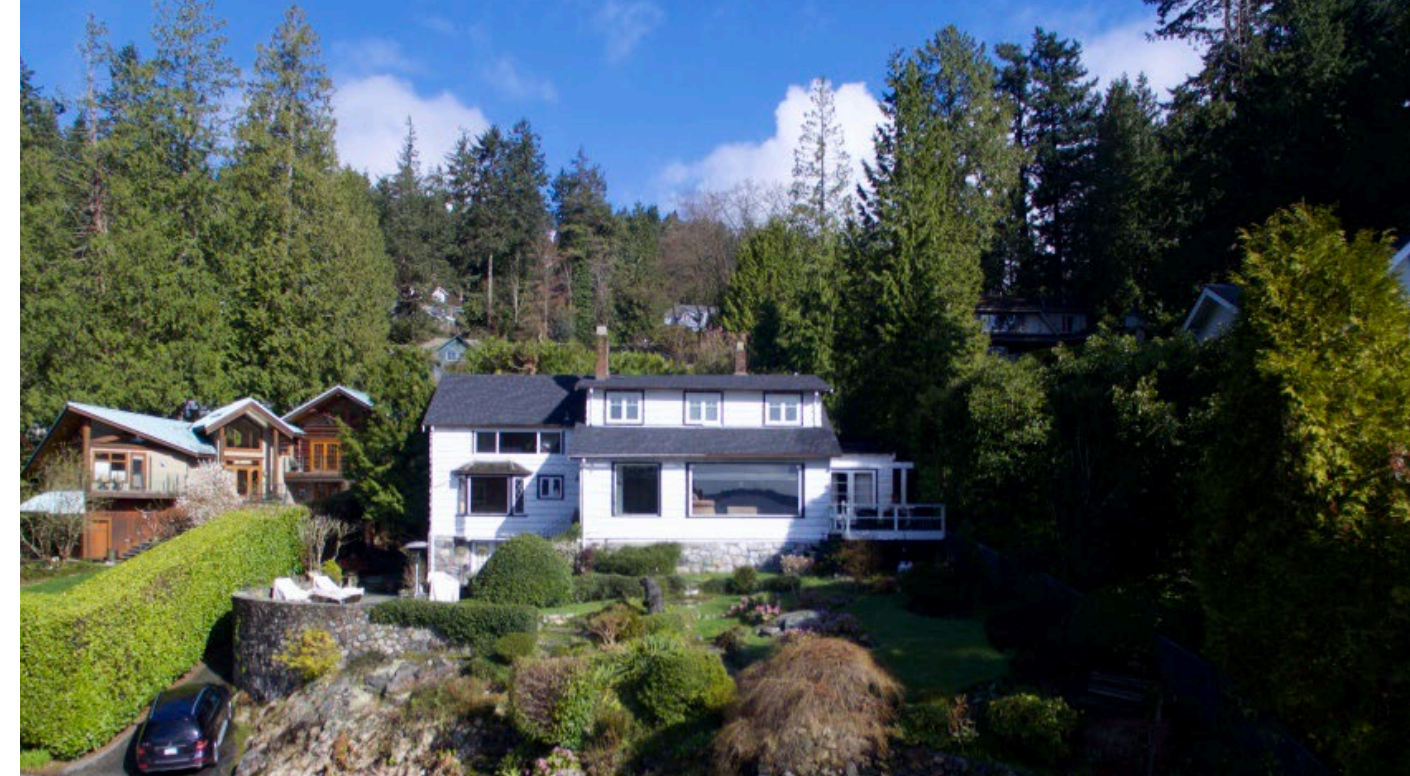
Image showing the current house at 4777 Pilot House Road, in comparison to neighbouring houses. House is in poor condition with limited heritage value.
