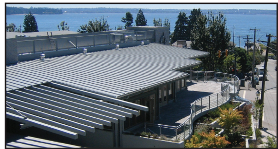
Rooftop mechanical systems screened and integrated into building design
