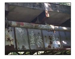
chipping. The process was difficult, costly, and required a crew gaining access by rope. New delamination could manifest at any time, requiring further expensive remediation.
