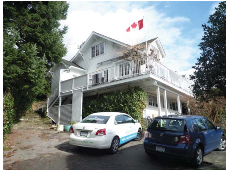
FRONT (SOUTH WEST)
