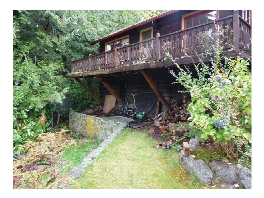
EXISTING RETAINING WALL WITH ROTTEN BALCONY ABOVE
