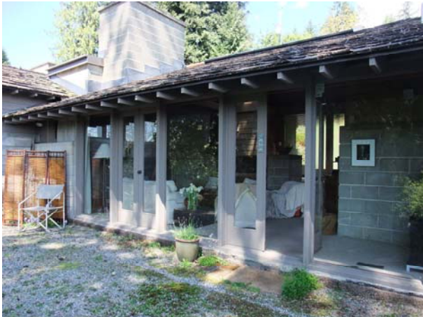
South-Facing Patio Doors to Living Room
