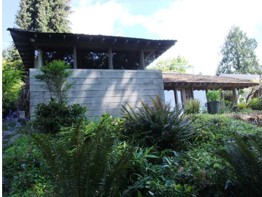
BOYD HOUSE ( viewed from south )
