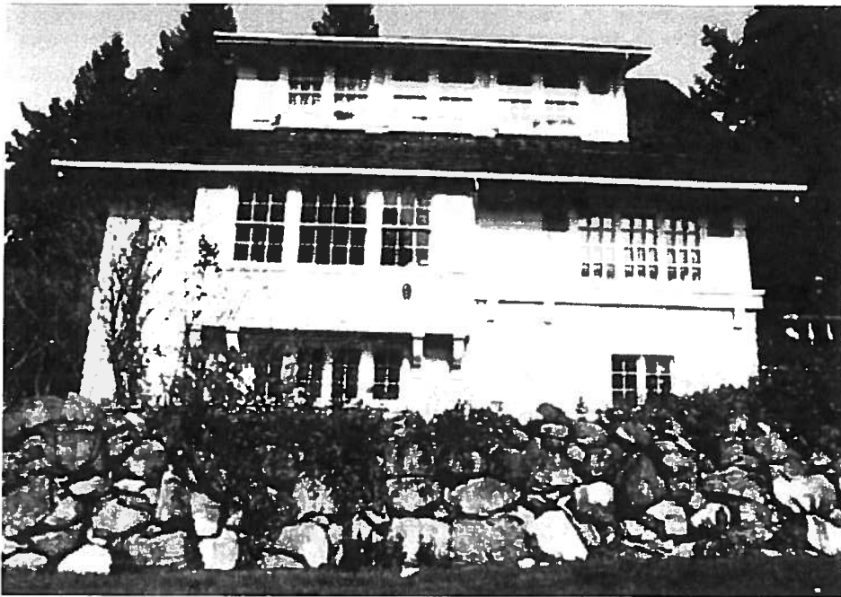
3321 Radcliffe Avenue in 1988. source: West Vancouver Archives 2585-03.1.0012
