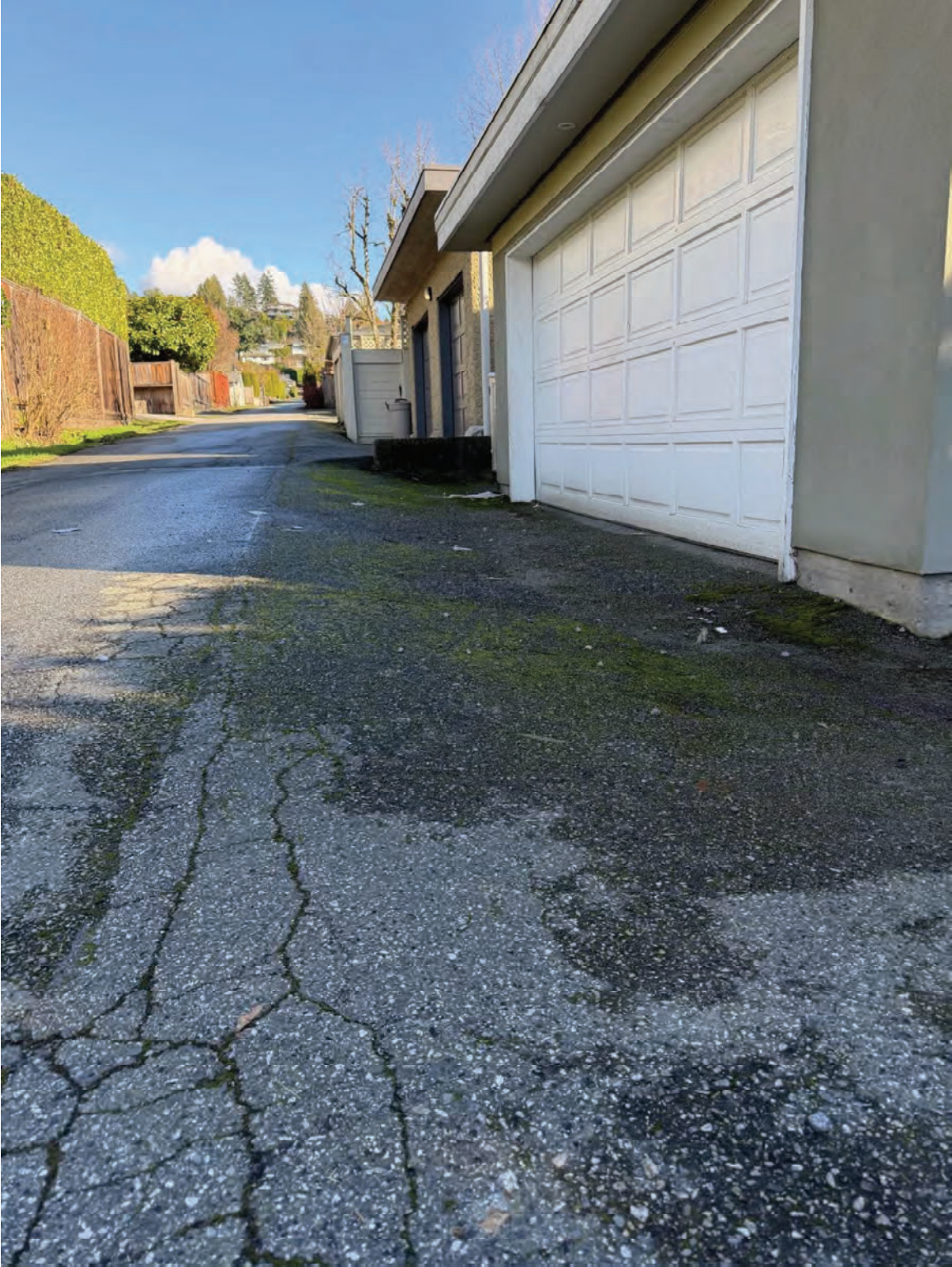
Existing garage entry condition and grade difference
