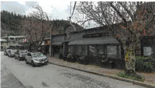
4 | NW CORNER OF SITE
